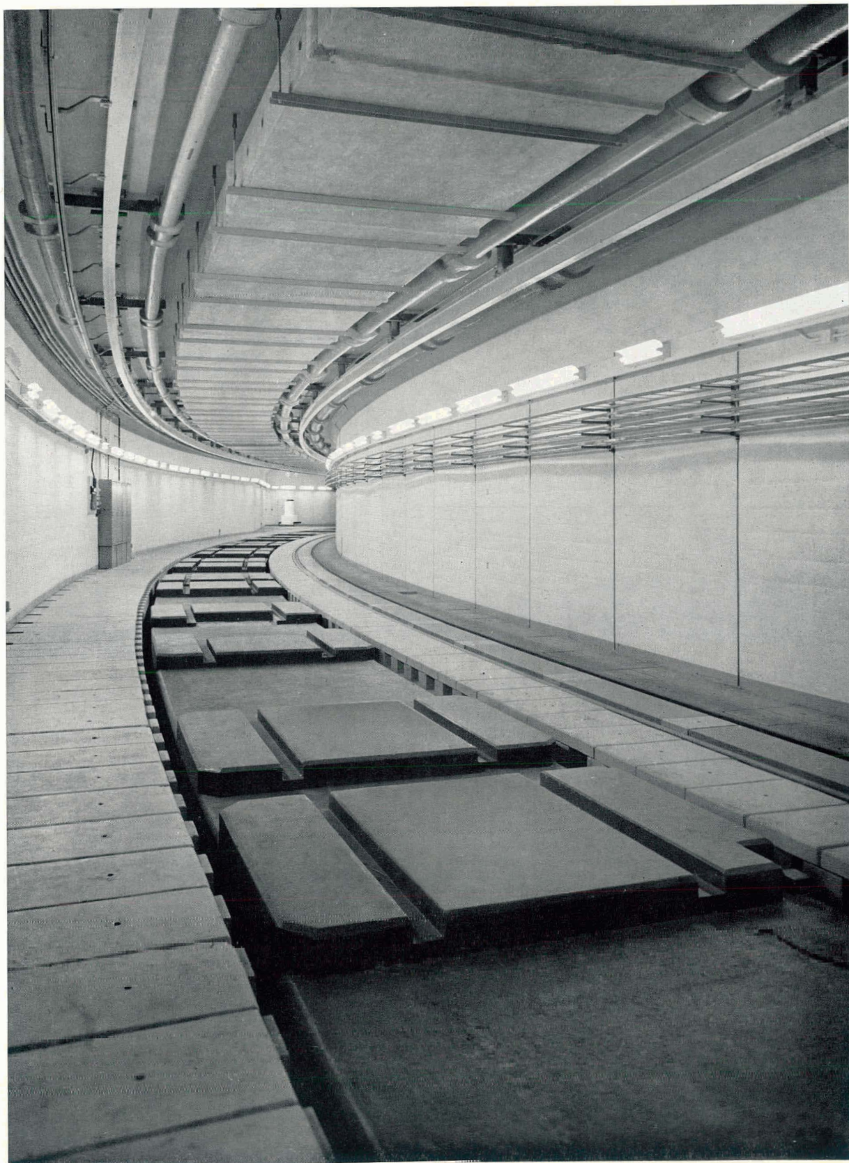
Interior of the ring building of the Eurotron, 25 GeV proton synchrotron.
