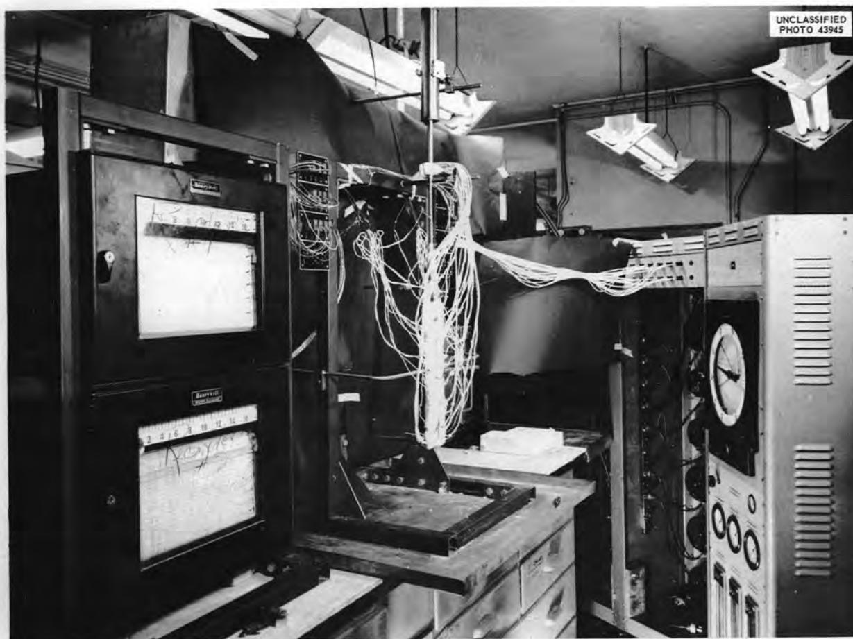
Fig. 166. MSR Convection Loop Mockup with External Resistance Heaters Installed.
