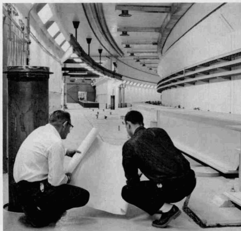
Figure 3. Inside the magnet tunnel looking toward the Cockcroft-Walton assembly. A portion of the platform on which the magnet will be mounted is visible. The upright cylinder at left front is one of the survey monuments.
