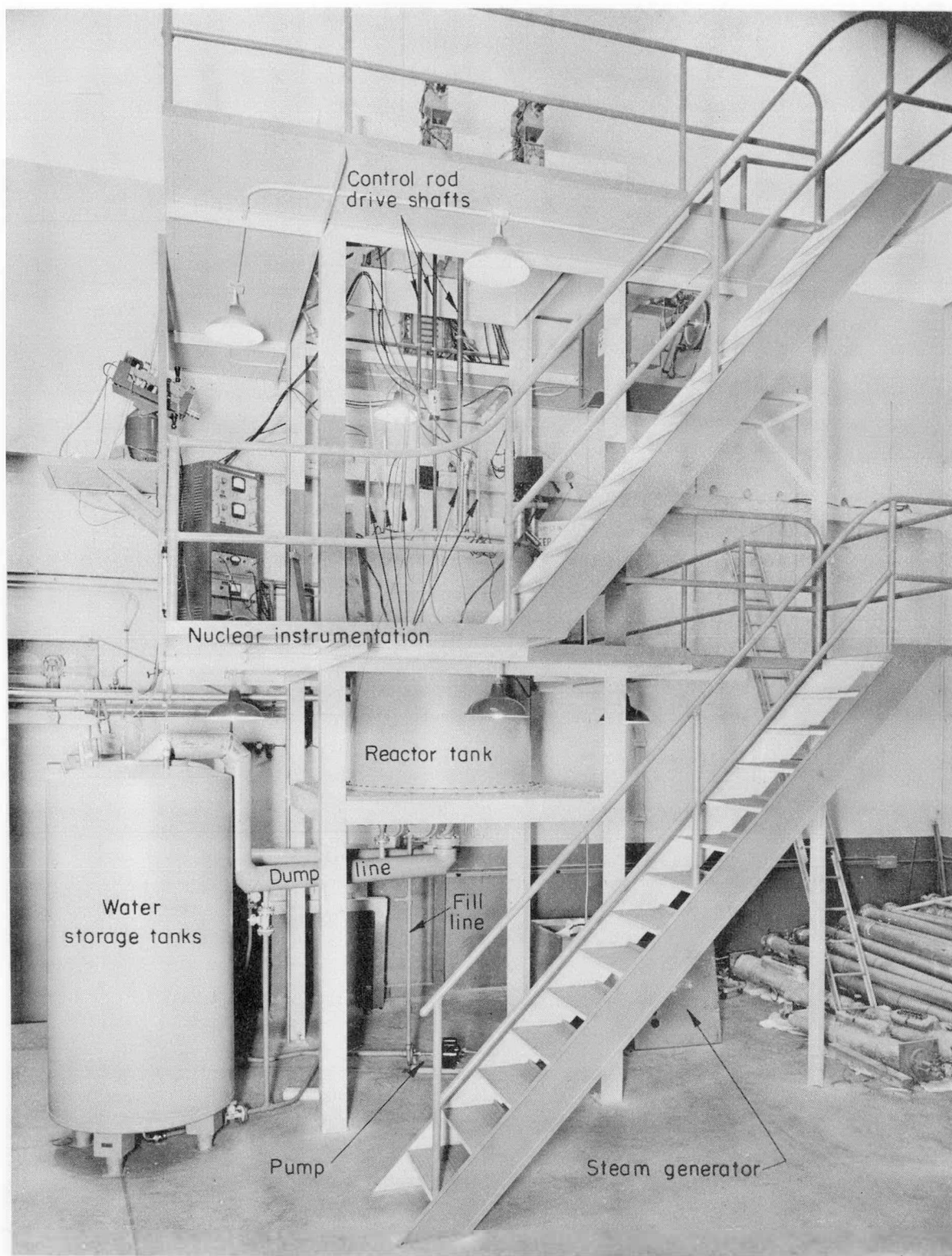
FIGURE 1. CRITICAL-ASSEMBLY STAND SHOWING MAJOR COMPONENTS
