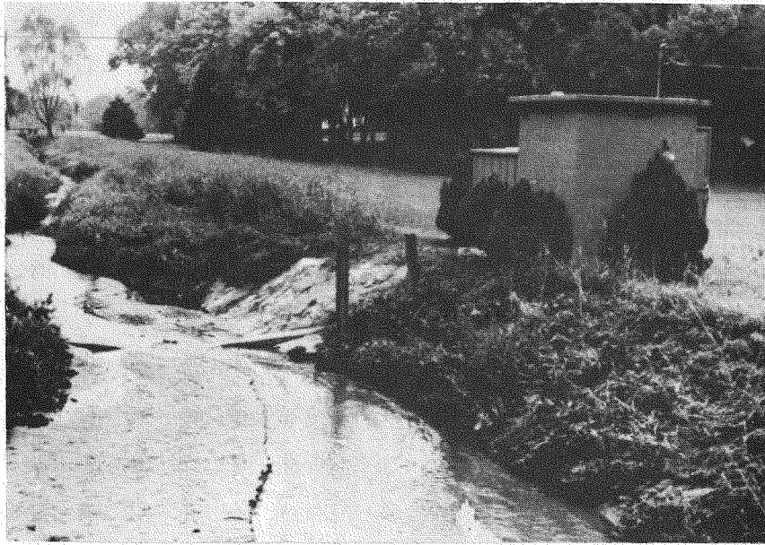
Figure 30. USGS gage house adjacent to Third Fork Creek.
