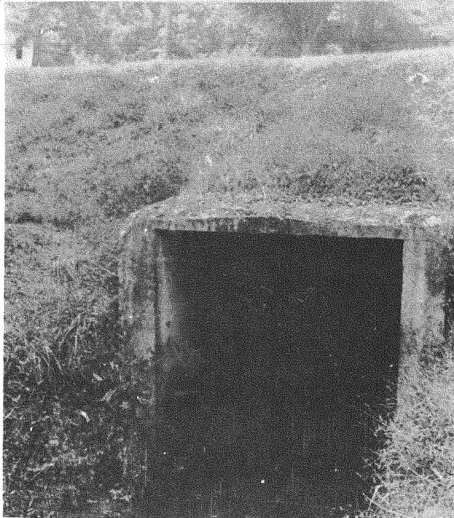
Figure 21. Culvert in Sub-basin W-1.
