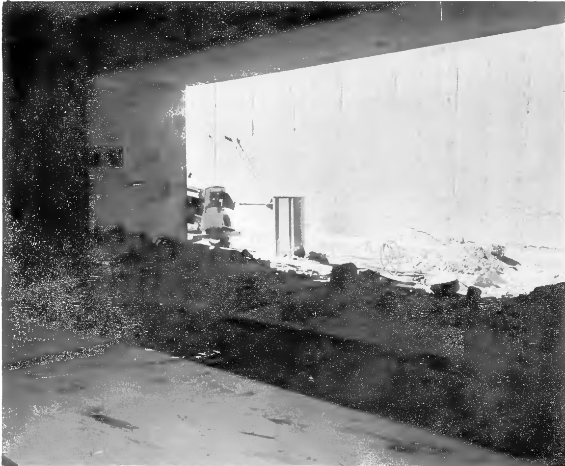
Fig. 3.1-Cracks in ramp side wall opposite door. View from interior of garage through door opening (postshot).
