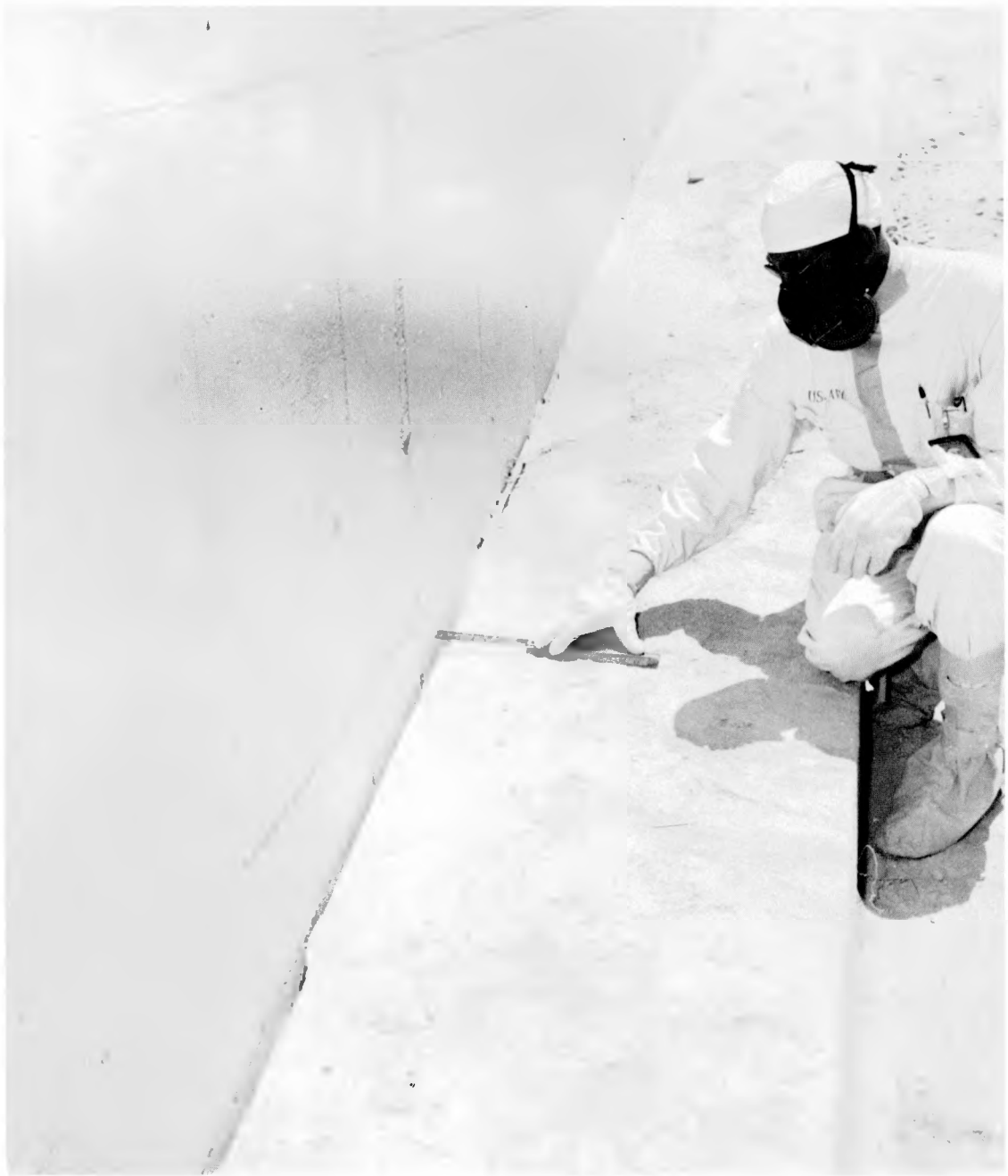
Fig. 3.2-Open joint between ramp slab and wall of main garage structure (postshot).
