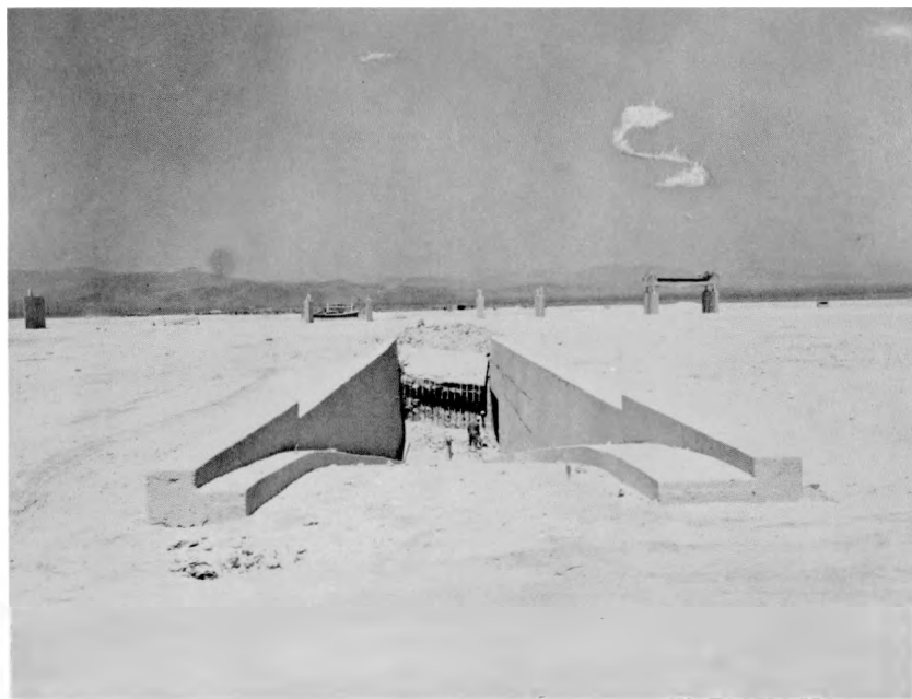
Fig. 3.4-View of ramp looking toward damaged end wall (postshot).
