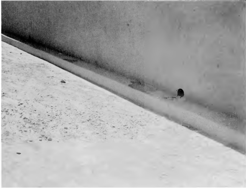
Fig. 3.3-Gravel backfill at weepers (postshot).
