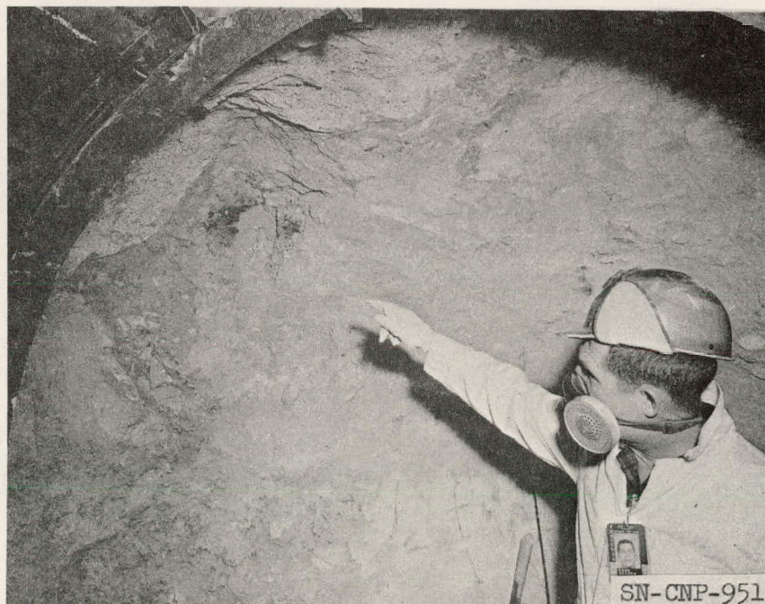
Fig.4. Fused material in U12-B Exploratory Drift.
