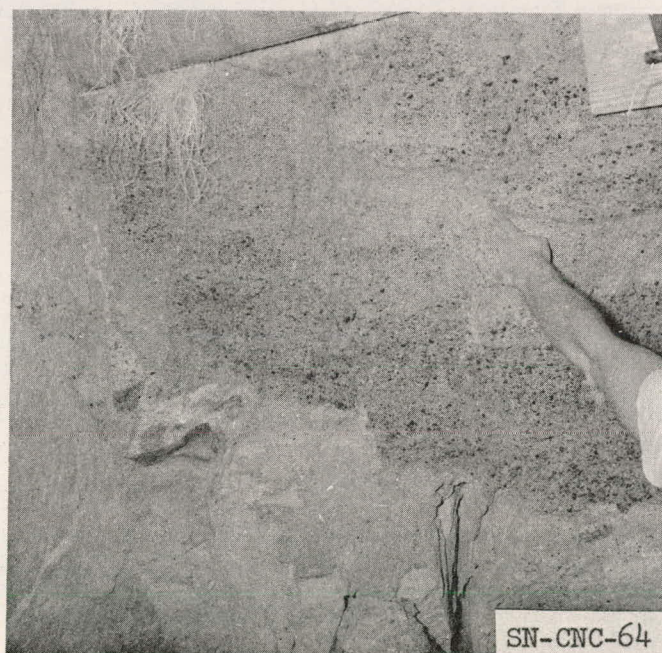
Fig. 12. U12-B "Raise" Drift (station 3+31 to 3+35). Open fractures in the massive lapilli tuff (TOS 7-8r ) are closed and curved on projection through the loose pebbly tuff (TOS 7-9r ).
