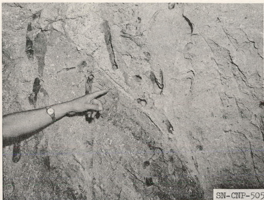
Fig.5. Collapsed TOS 7-7r showing shear plane in U12-B Exploratory Drift.
