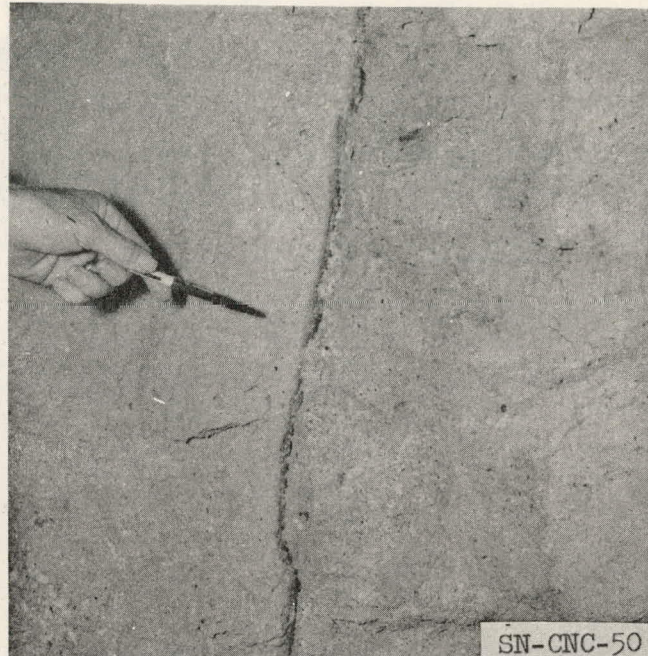
Fig. 7. Stringer of fused rock and adjacent crushed TOS 7-6r (right) and collapsed TOS 7-7r (left) at station 16+25 in U12-B Exploratory Drift.
