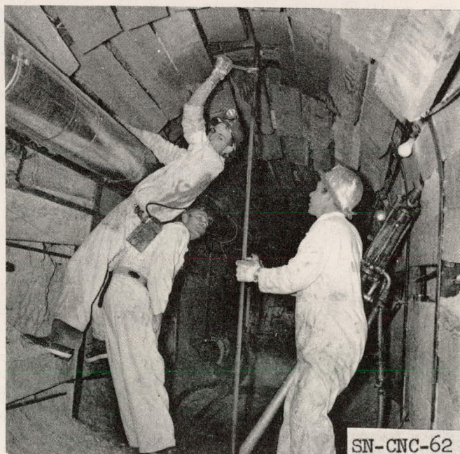
Fig.20. Cavity probe operation over station 3+20 in U12-B "Raise" Drift.
