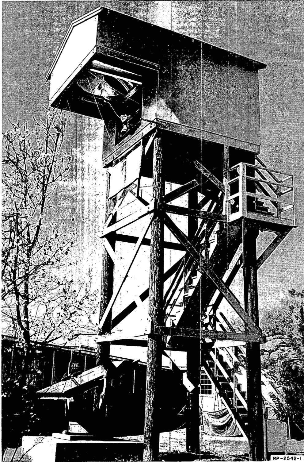
FIG. 1 SOLAR FURNACE AT STANFORD RESEARCH INSTITUTE
