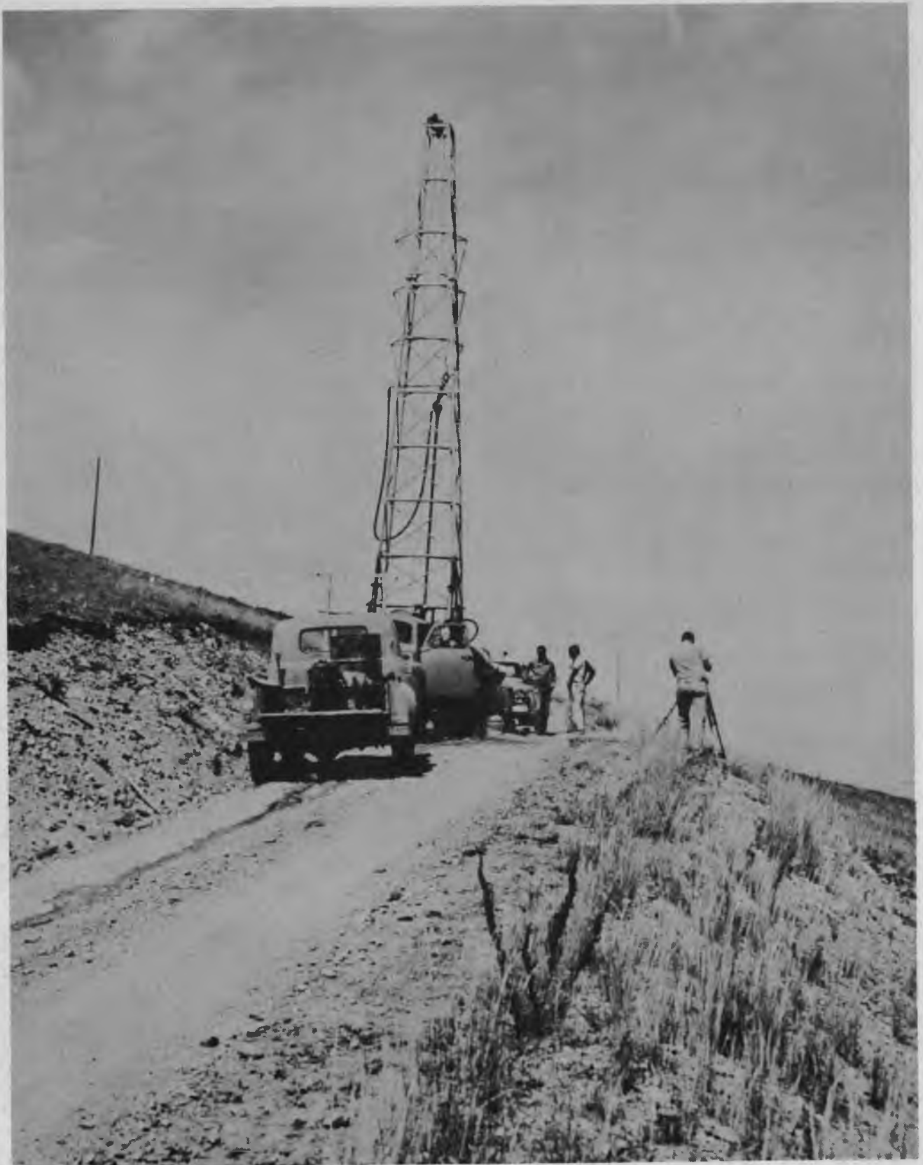
Fig. VIII-1. Core Drilling Rig and Drill Crew on Location at the Site. Part of Survey Team with Transit Shown at Right
