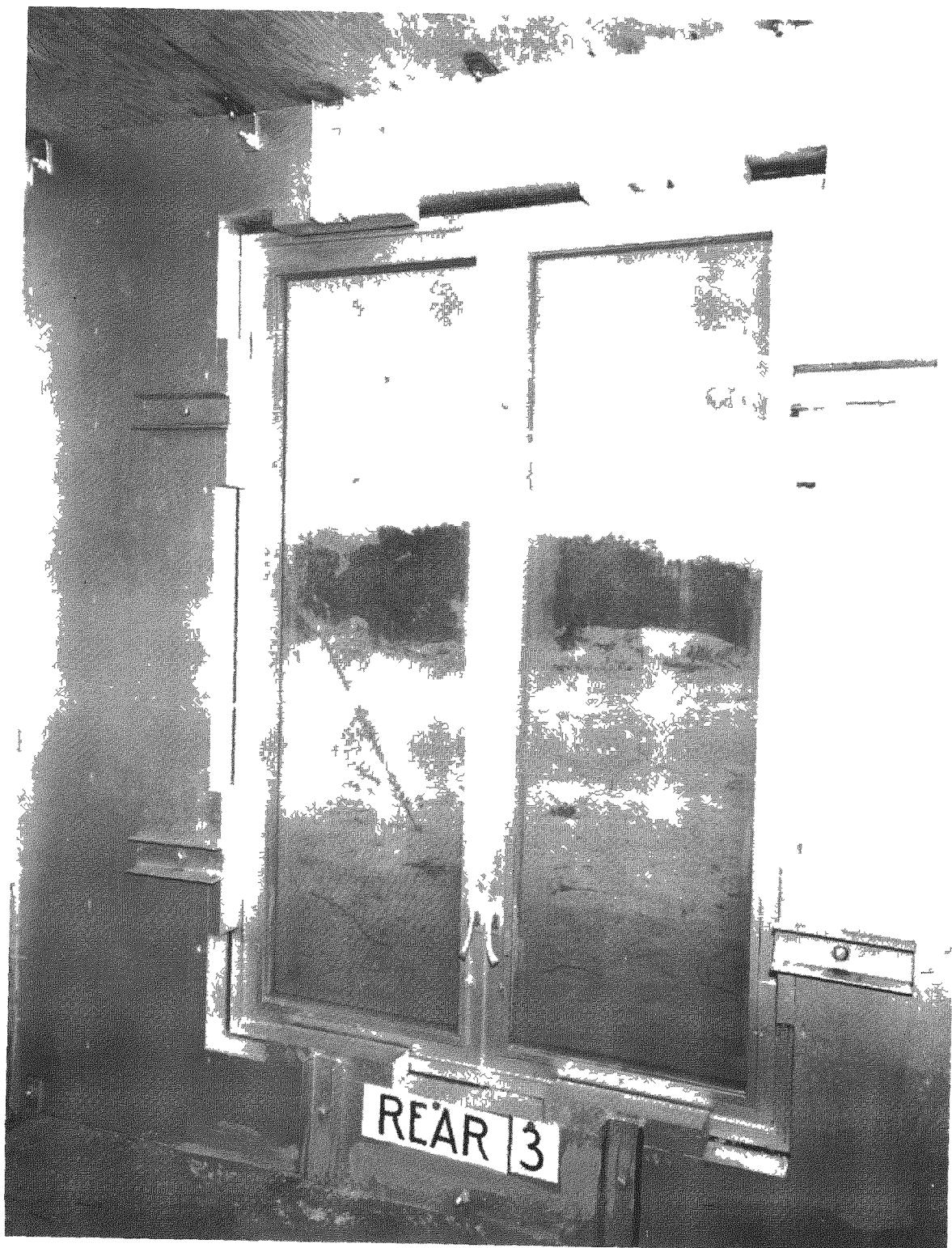
FIG 347 Inside of Casement Window 13 before the Blast This window was a duplicate of window 5 with wire glass on the left and tempered glass on the right
