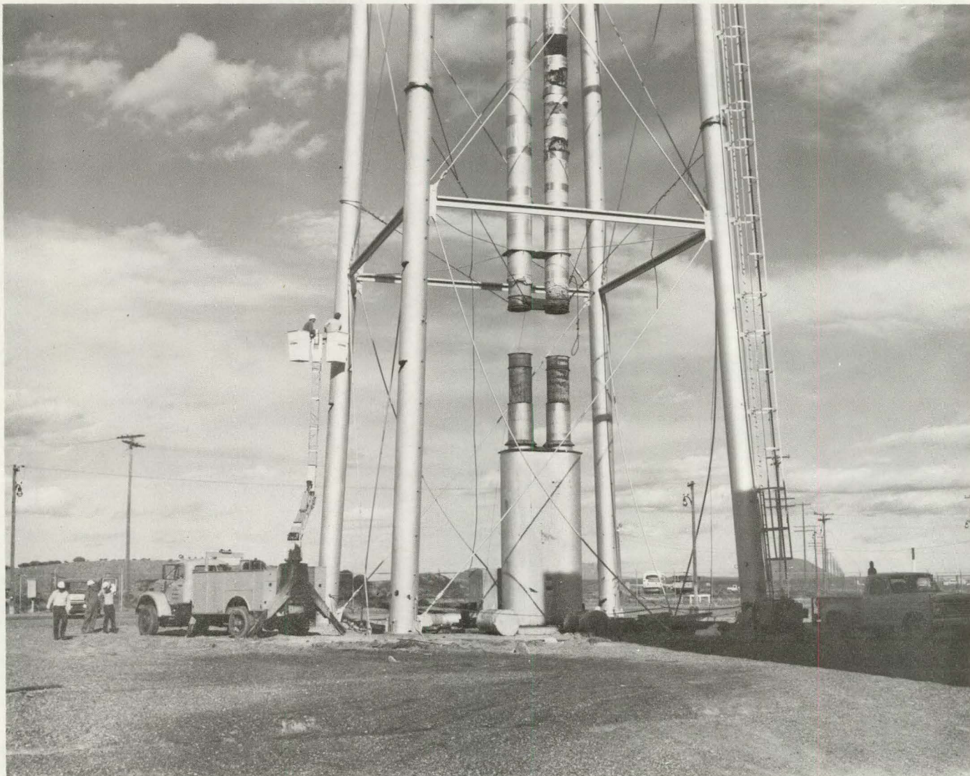
Fig. 4 View of the OWR showing removed sections of the inlet and outlet piping.
