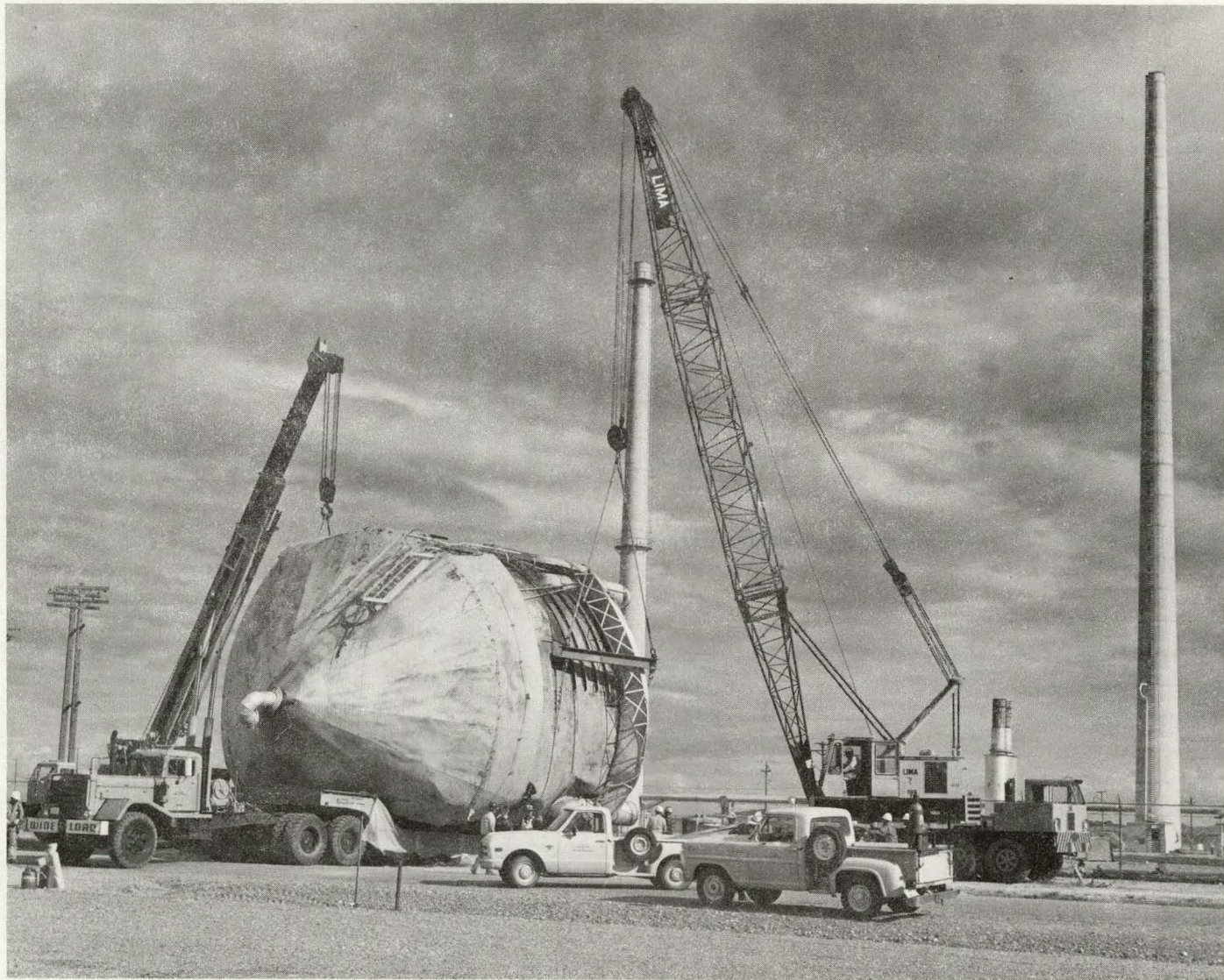
Fig. 10 View of the OWR being loaded for transportation.
