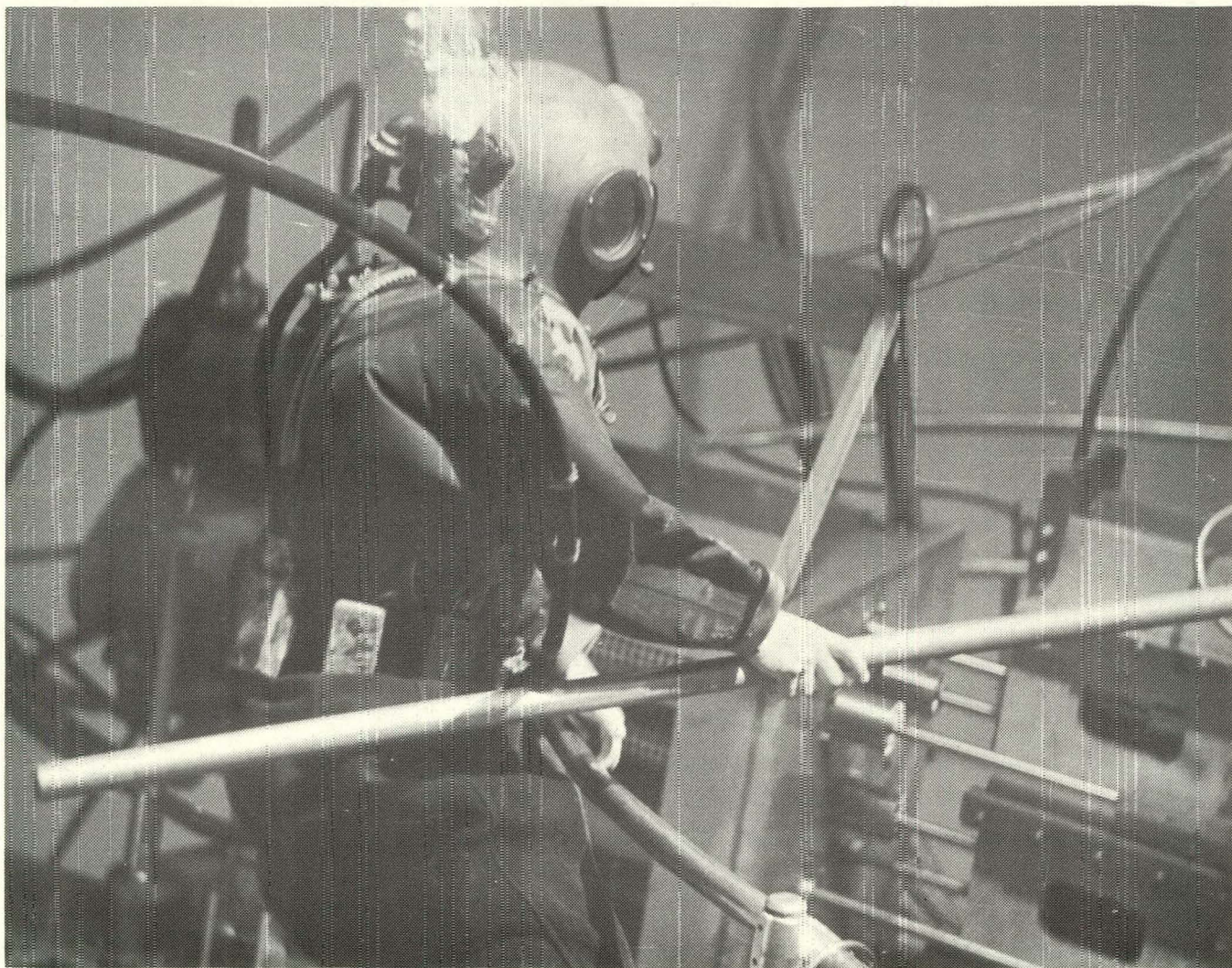
FIGURE V-4. GCRE-I FLANGE BOLT TIGHTENING OPERATION
