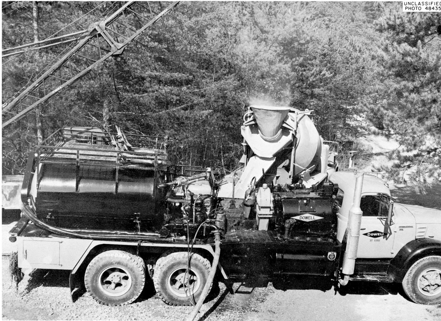
Fig. 1.57. High-Pressure Pump Truck and Bulk Dry Cement Carrier Used in the First Fracturing Experiment.
