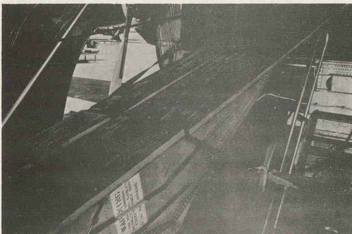
Figure B-93 Nylon safety straps used to prevent slippage of the shoring while loading mockup
