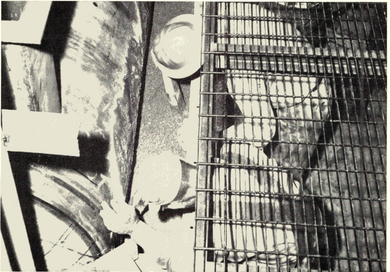
FIGURE 15. - Placing of Insulation Around the Electrolyte Chamber.
