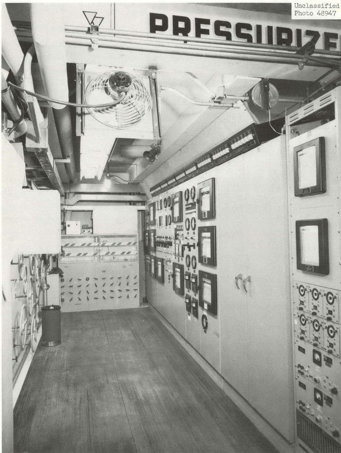
Fig. 46. Operating Area for ORR Pressurized-Water Loop. Control valve handles at left, instrument panel at right, and water sampling station in background.
