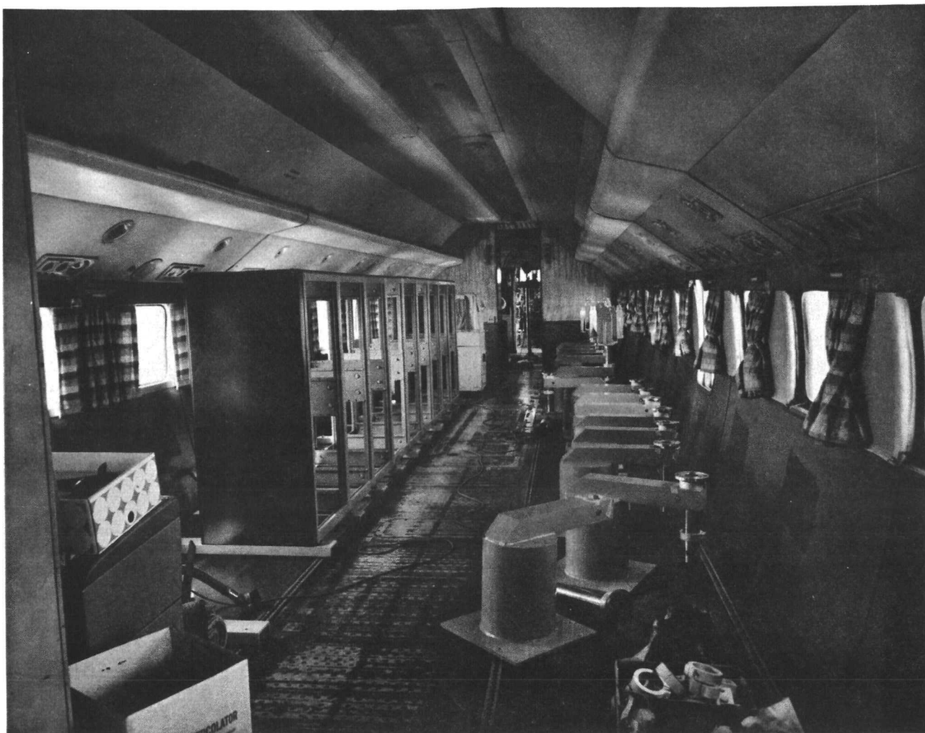
Figure 16. Electronic Racks in Aircraft. Looking forward, the empty racks as shown during the installation. They are bolted to the seat rails.
