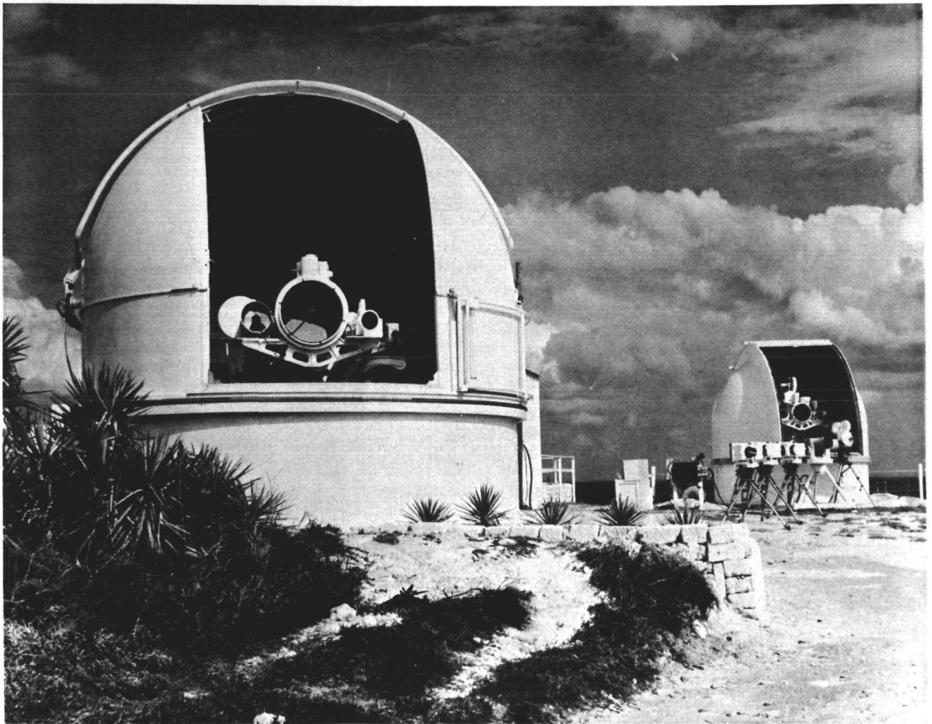
Figure 1. LA-24 and ME-16 Tracking Mounts at Bermuda. The LA-24 is shown on the left.
