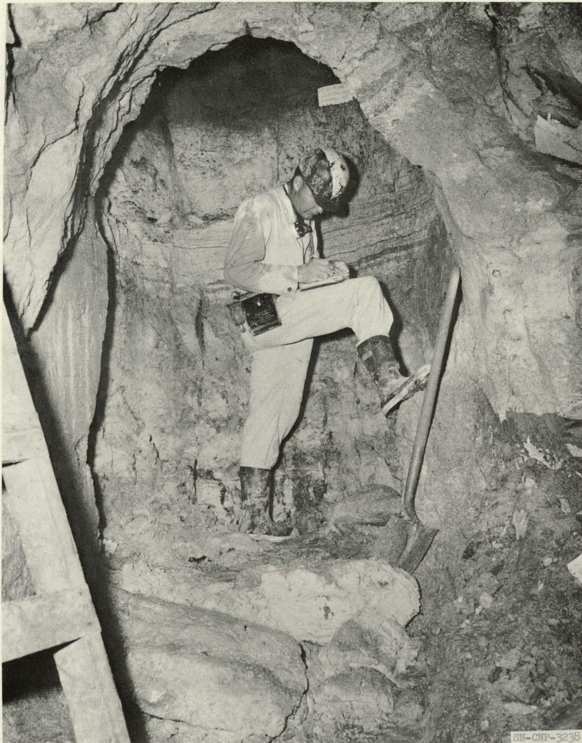
Fig. 5. Lower 2/3's of Hobo Shot 14A cavity after rubble was removed. Cavity about 5 ft in diameter and 11 ft high. Note vertical fractures on either side of geologist's left leg. Subunit V begins just above his waist.
