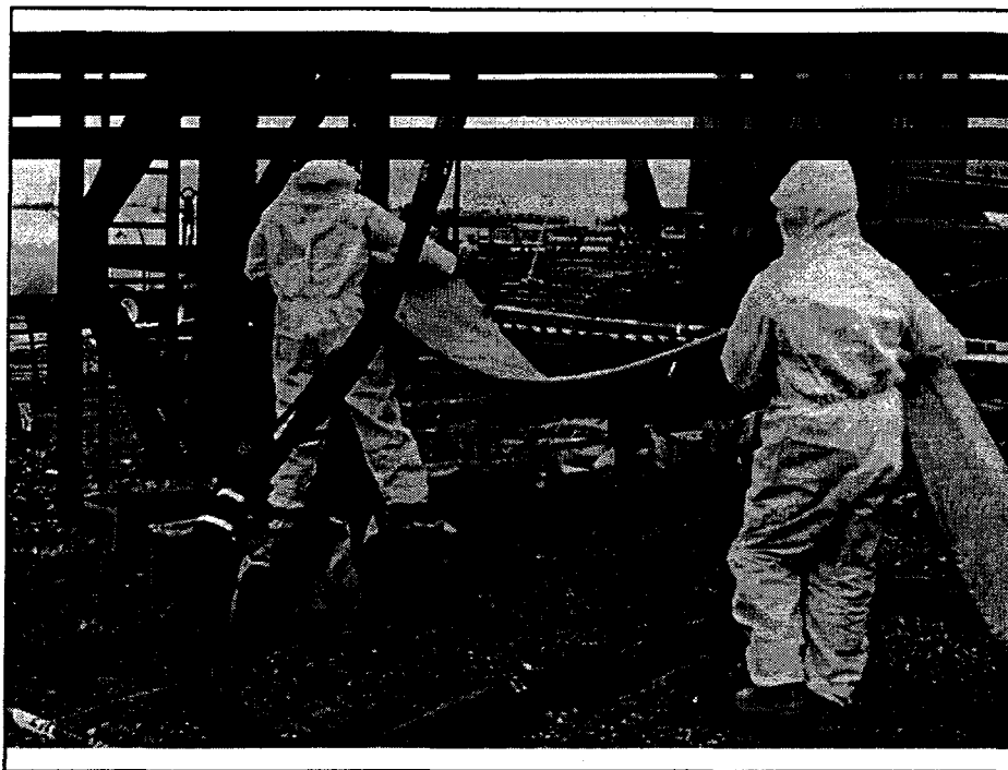
Figure 3. Wicks being installed in hollow mandrel.
