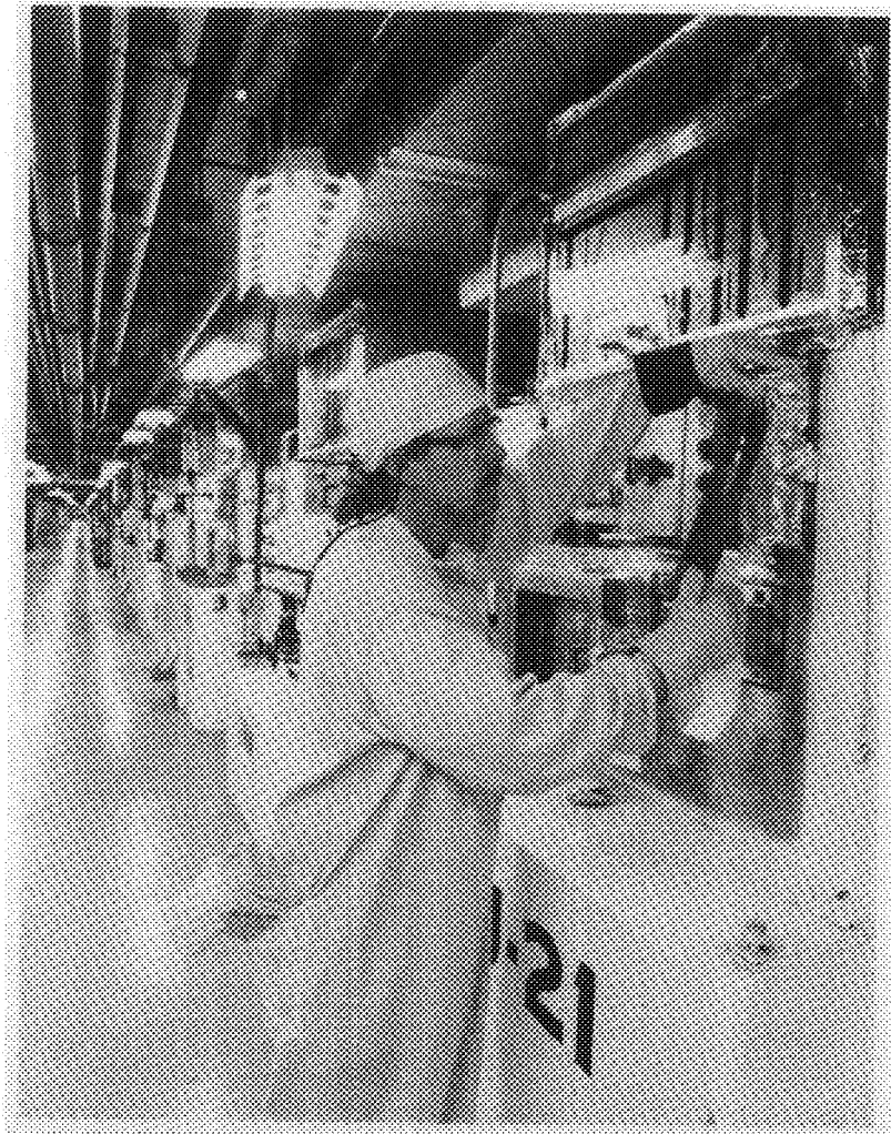
Figure 22. Waste is Packaged out of PUREX N-Cell, as Part of Deactivation, 1996.
