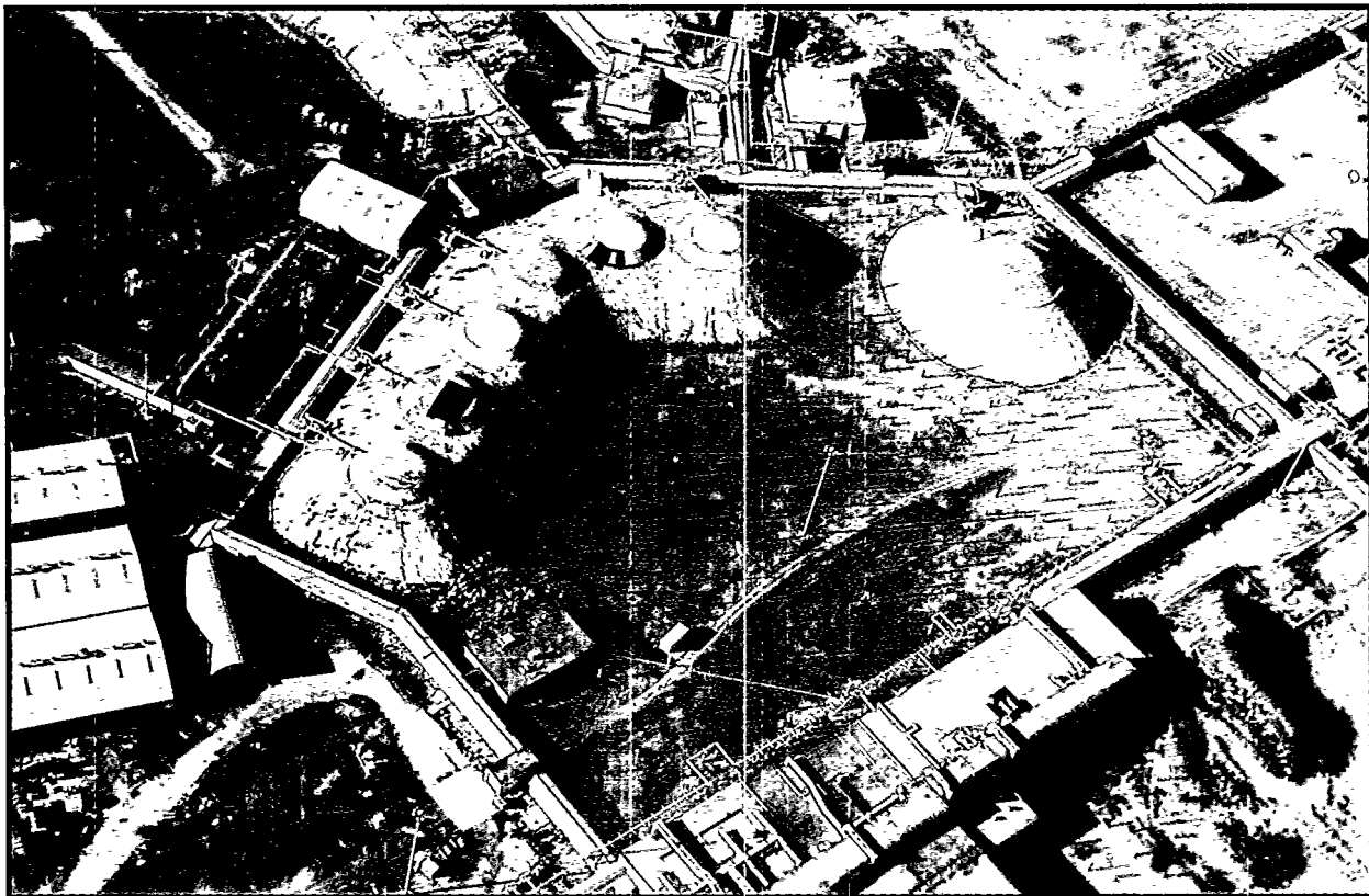
"Gravel Gerties" are circular concrete structures whose roofs consist of cable mesh supporting large amounts of gravel. Beneath them are bays, where workers assemble and disassemble nuclear warheads. Should a warhead's conventional explosives accidentally detonate, the roofs of these structures are engineered to give way, releasing the gravel and trapping the plutonium particles. Up to 2,000 warheads per year are now being dismantled at this site. Pantex Plant, Amarillo, Texas. November 18, 1993.
