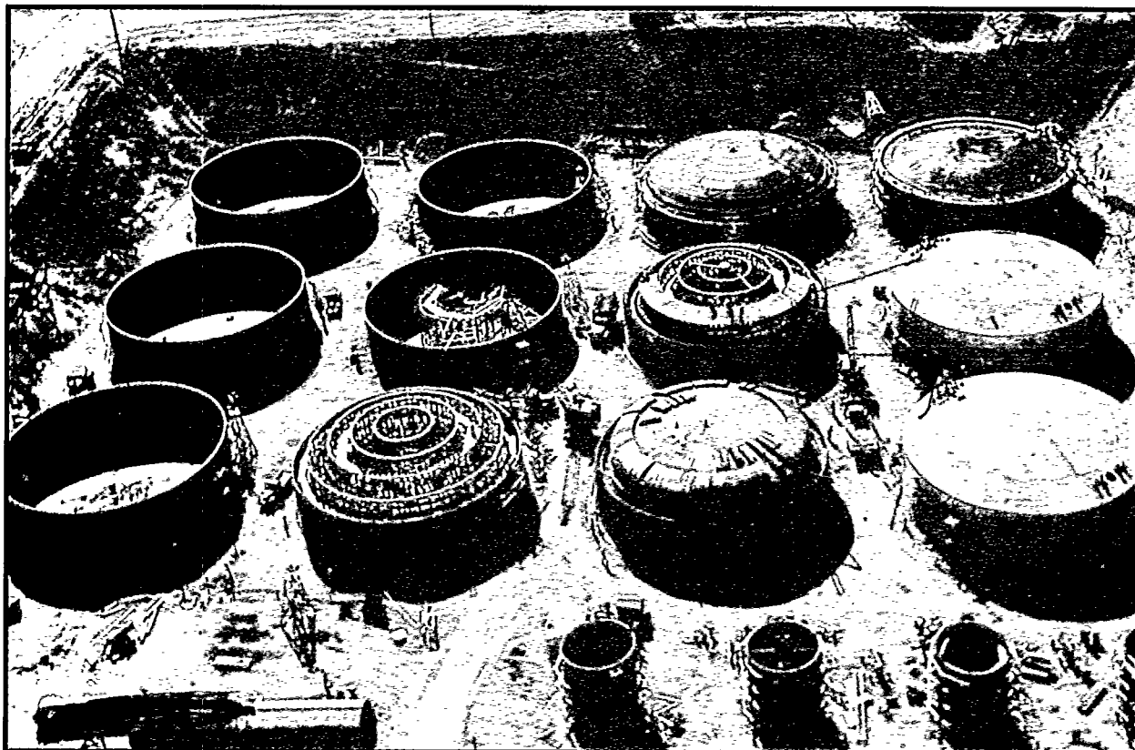
These single-shell tanks stored high-level radioactive wastes from Hanford's chemical separations plants. The tank farm shown here was built for the Manhattan project during World War II to hold wastes from the T Plant, which separated plutonium from irradiated reactor fuel. 200 Area, Hanford Site, Washington. Mid-1944.
