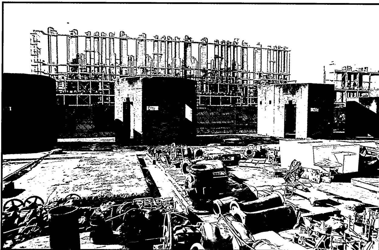
Savannah River Heavy Water Plant being dismantled. The plant separated and concentrated the small fraction of deuterium found in ordinary water to produce "heavy water." Heavy water produced here between 1952 and 1982 was used in plutonium and tritium production reactor on the site and in nuclear weapons. Heavy Water Extraction Facility, Savannah River Site, South Carolina. January 8, 1994.
