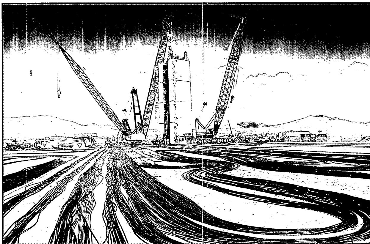
Signal cables laid out on the desert floor at Yucca Flat. These cables relayed scientific data to recording trailers on the surface as the nuclear device detonated deep underground. The tower above the emplacement hole was used to assemble a package of scientific instruments in a canister attached to the nuclear device. The tower was dismantled before the detonation took place. Yucca Flat, Nevada Test Site. (No date available.)
