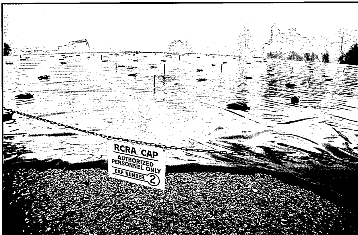
RCRA cap. Ten acres of black plastic cover a radioactive waste landfill in Oak Ridge. This high-density polyethylene cap is designed to prevent gases from escaping, reduce erosion, and keep rainwater from leaching contaminants into the groundwater. Installed in 1989, the cap is designed to last 15 to 20 years. Solid Waste Storage Area 6, Oak Ridge Reservation, Oak Ridge, Tennessee. January 10, 1994.
