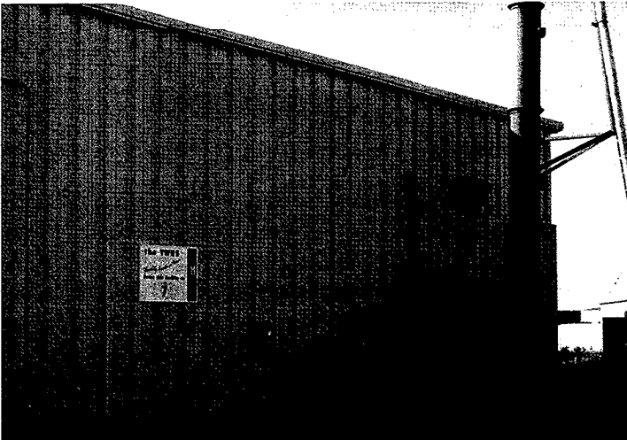
Figure 3-4. 213-W Dry Waste Compactor
