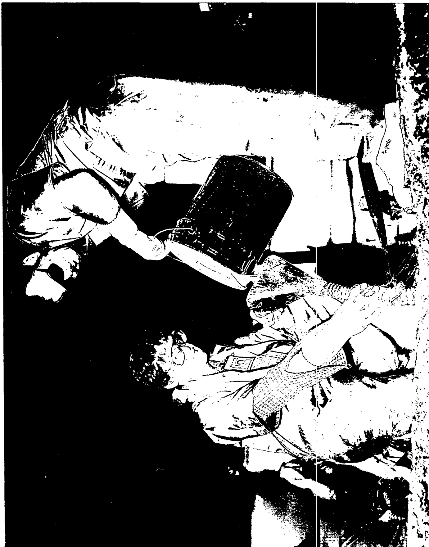
Figure 11. Application of BRISTAR (94-793-1-3).
