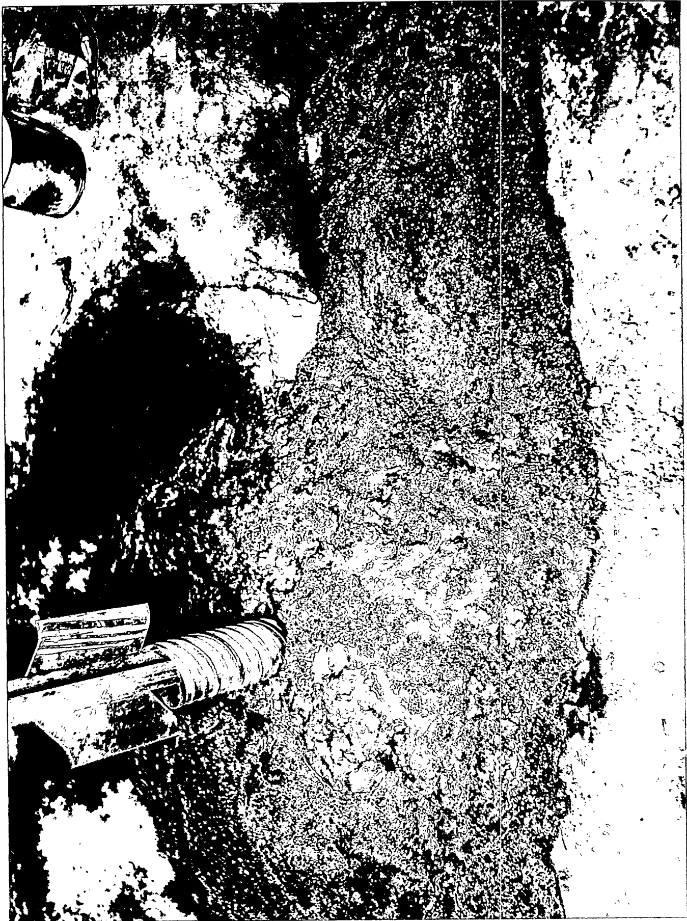
Figure 28. Grout/sludge emission from hole 6 during grouting of hole 2 (94-749-1-5).
