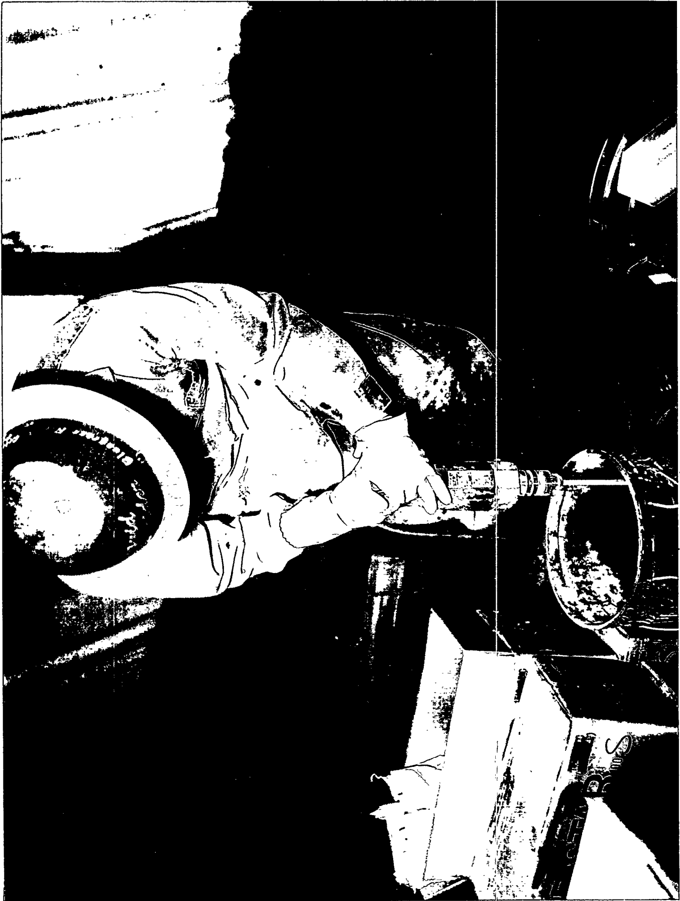
Figure 10. Preparation of BRISTAR (94-793-1-5).
