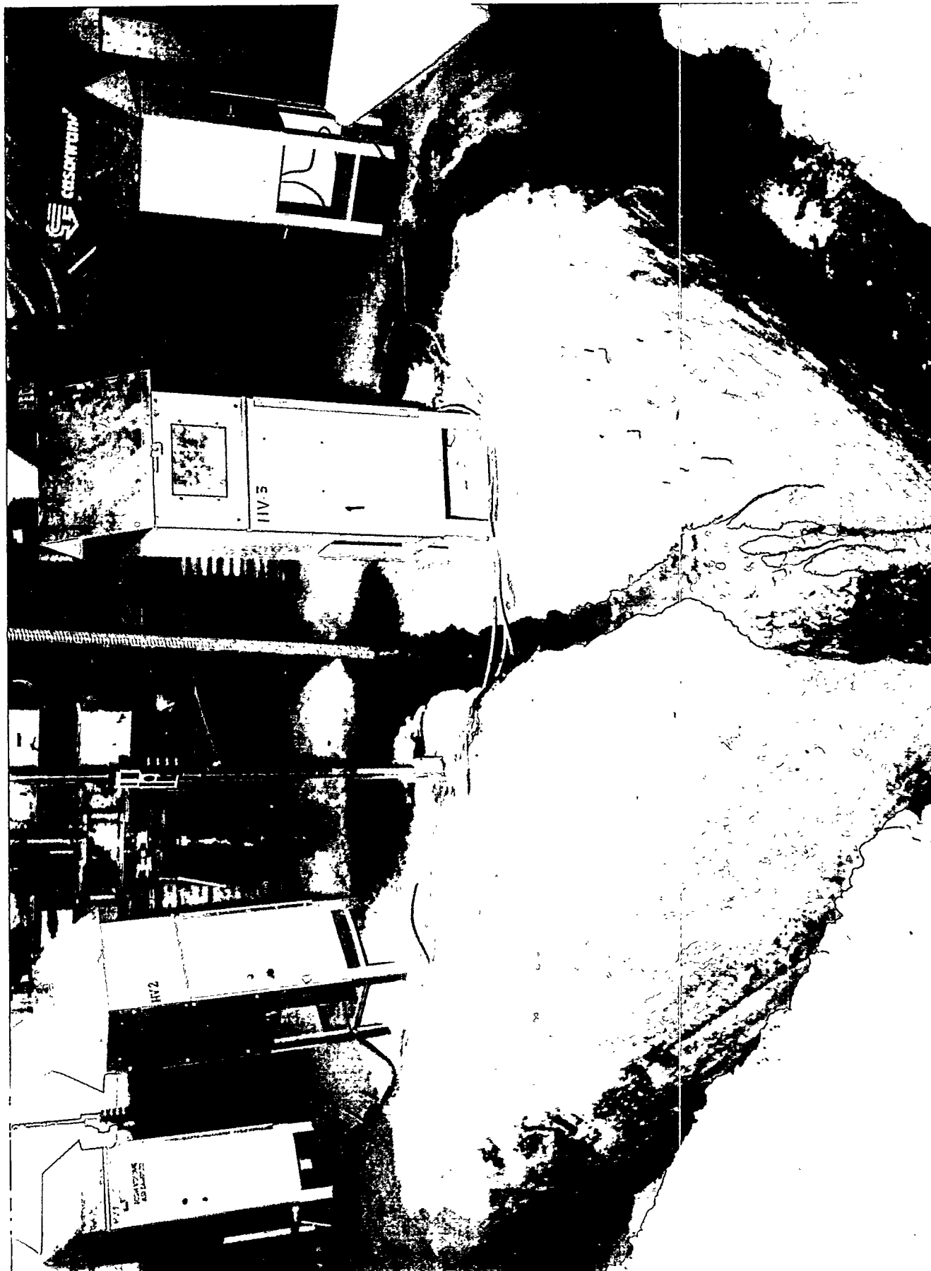
Figure 27. Grout collection pit during grouting (94-716-4-1).
