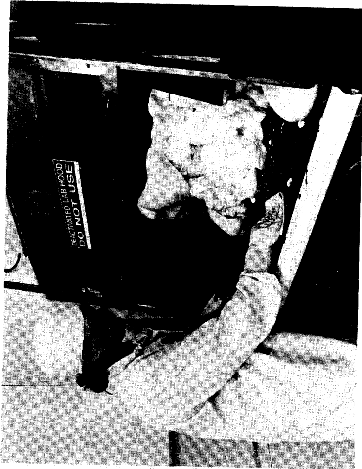
Figure 33. Foam is Spread Inside PUREX Laboratory Hood in Final Deactivation Step, 1996.
