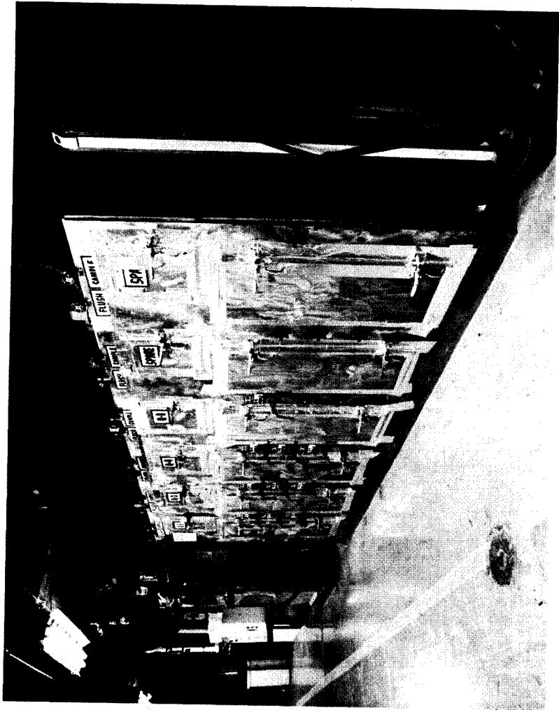
Figure 25. Q Cell Samplers Sealed Shut After Deactivation, PUREX Plant, 1994.
