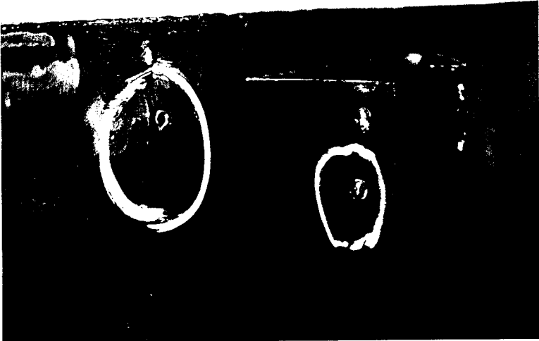
43-TU-02 - 1/4-inch Diameter Hole at Middle Riser Location:
