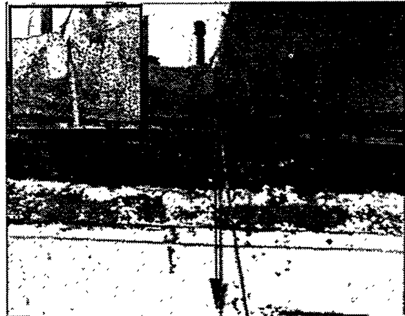
Figure 1. Diamond wire and cut line.
