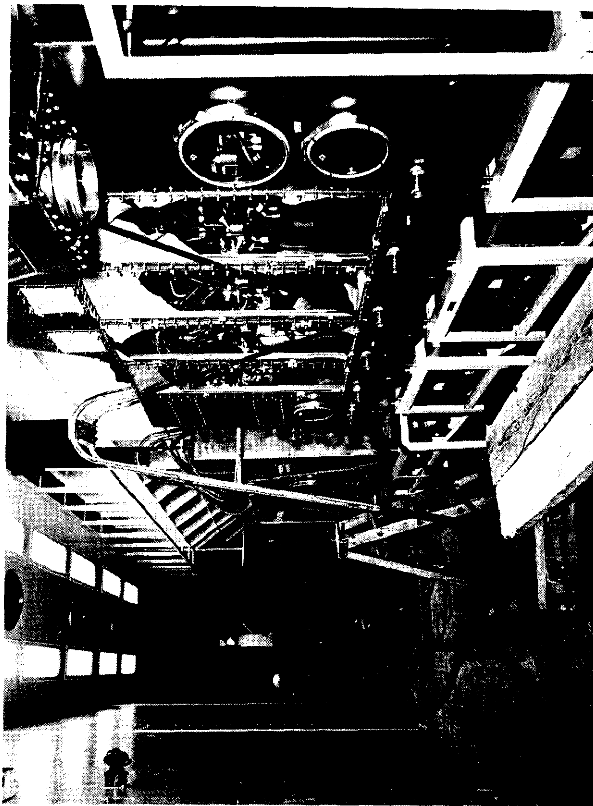
Figure 5-1. A-Line Installation, November 1950.
