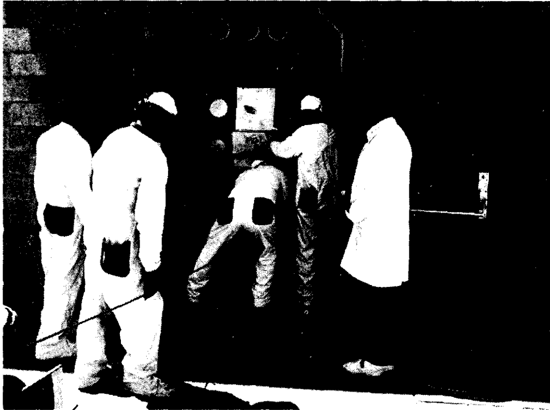
Figure 1-3. Removal of Plutonium Metallurgy Glove Box from the 231-Z Building During World War II.
