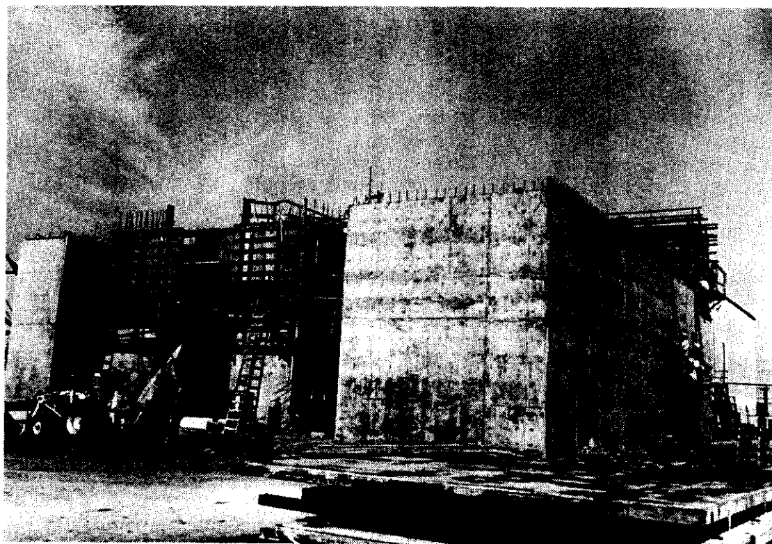
Figure 12-2. PRF Construction, October 1962.
