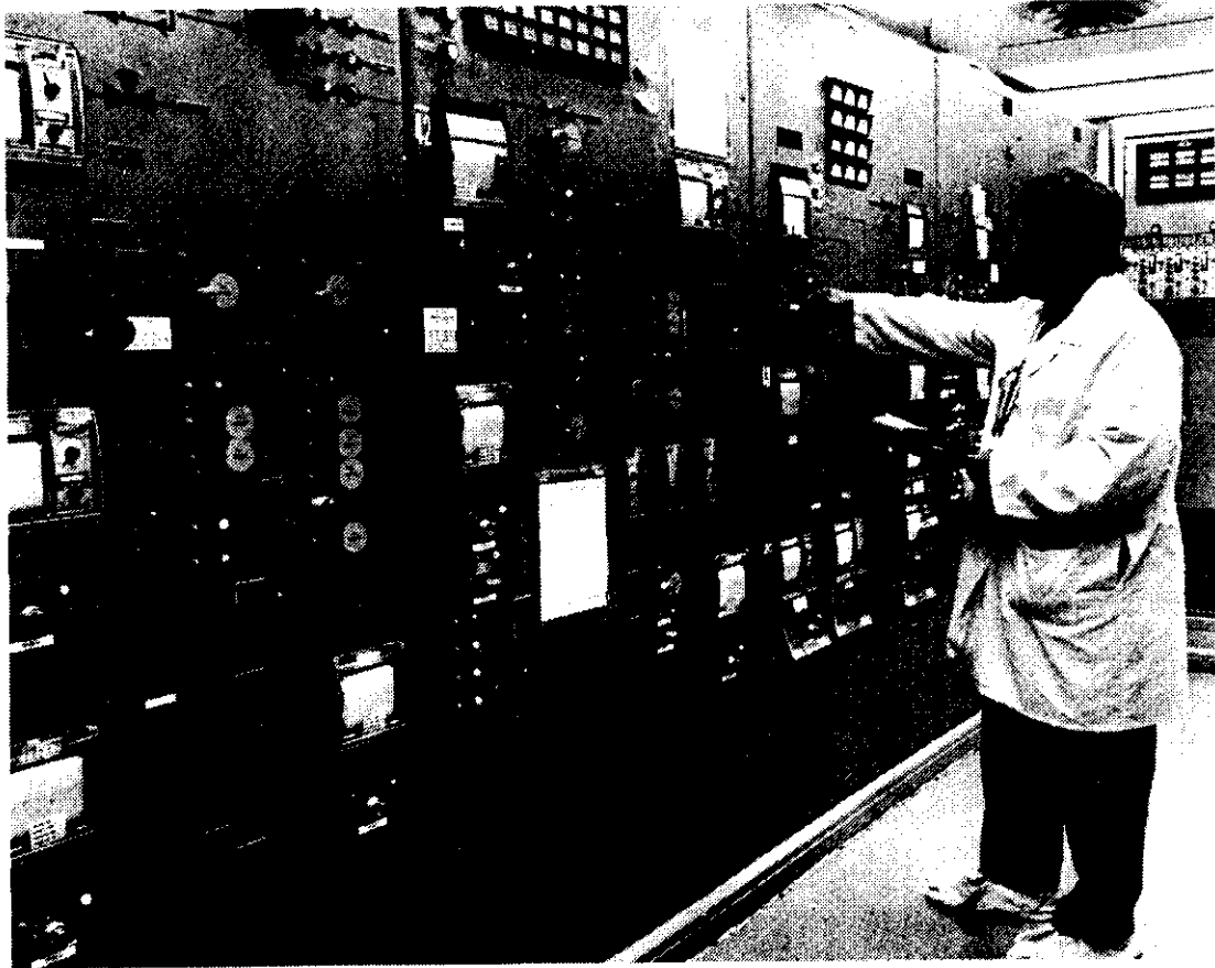
: Figure 12-7. PRF Control Room During Last Campaign, 1988.
