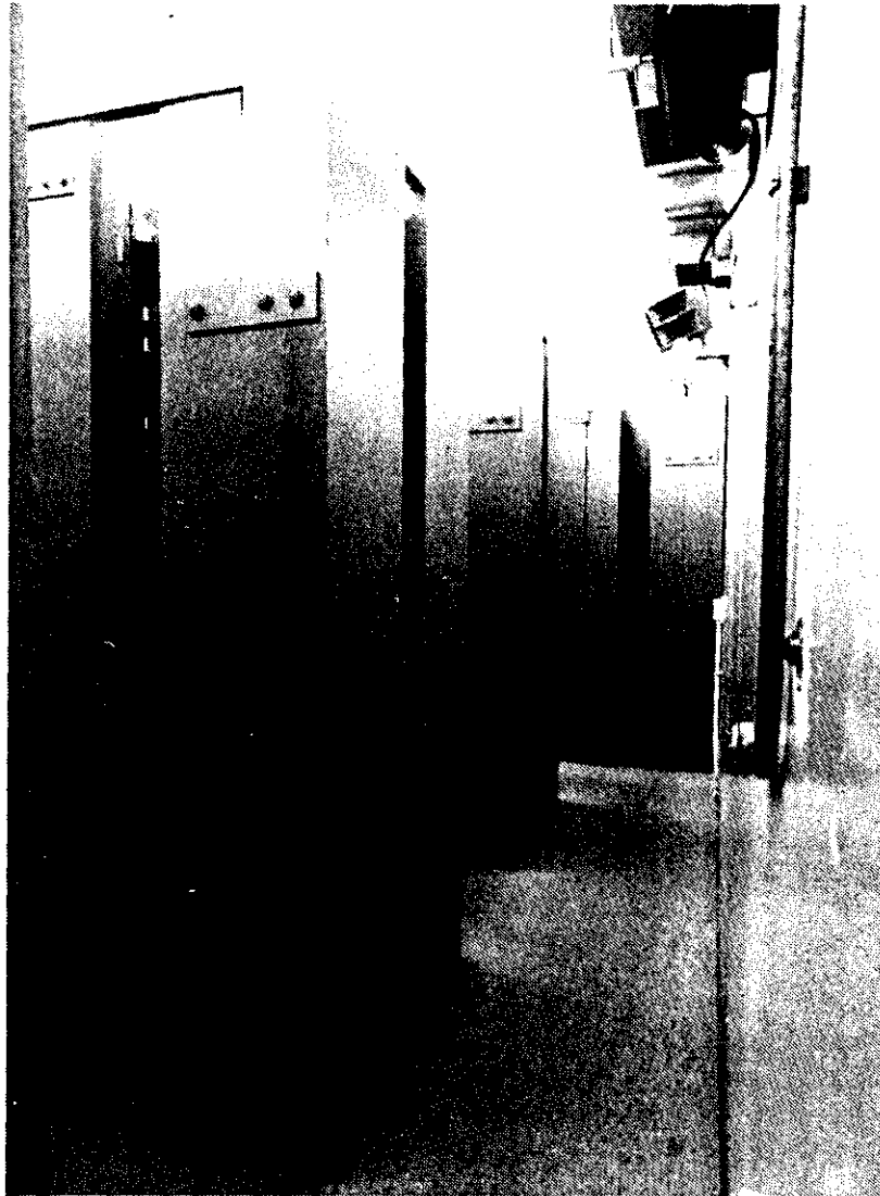
Figure 14-2. Plutonium Storage Vaults in the 2736-Z Facility, 1973.
