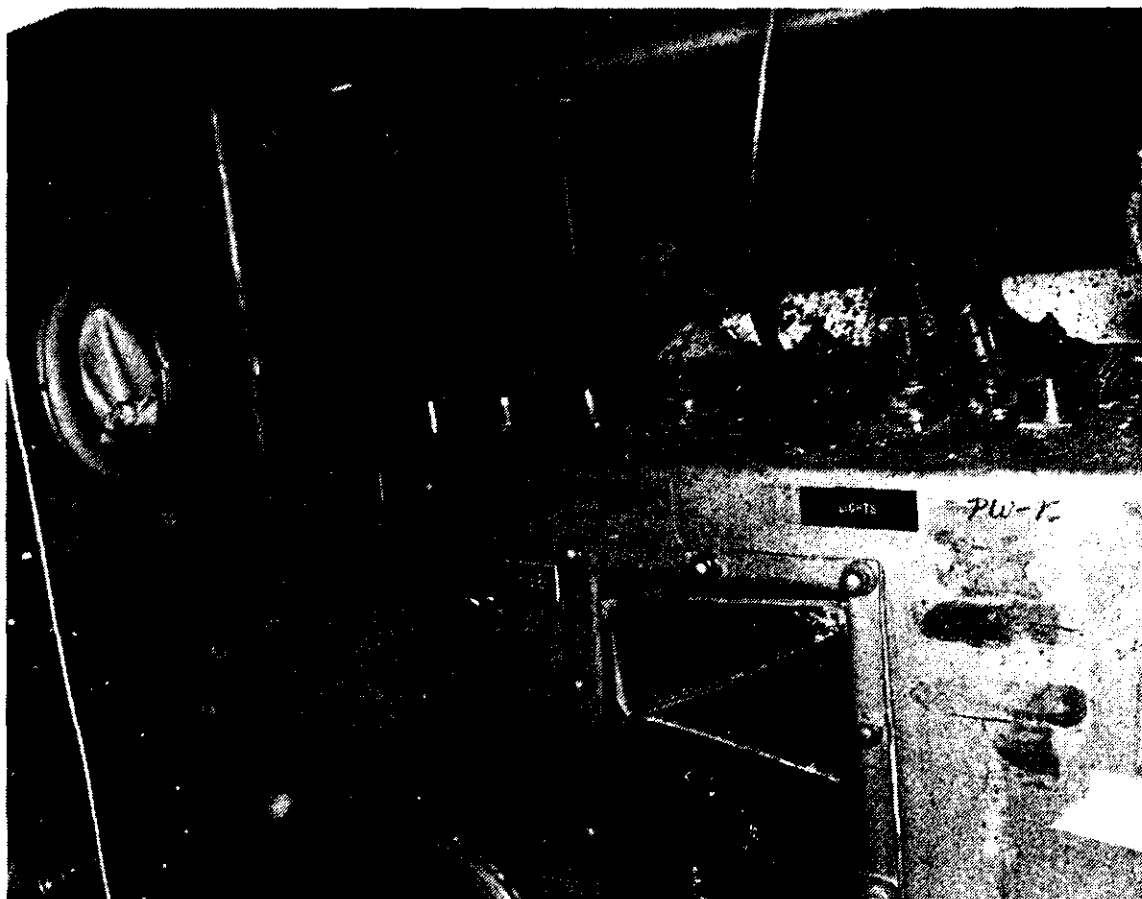
Figure 11-3. Hood Face Blown Out in Explosion, 242-Z Facility, August 30, 1976.
