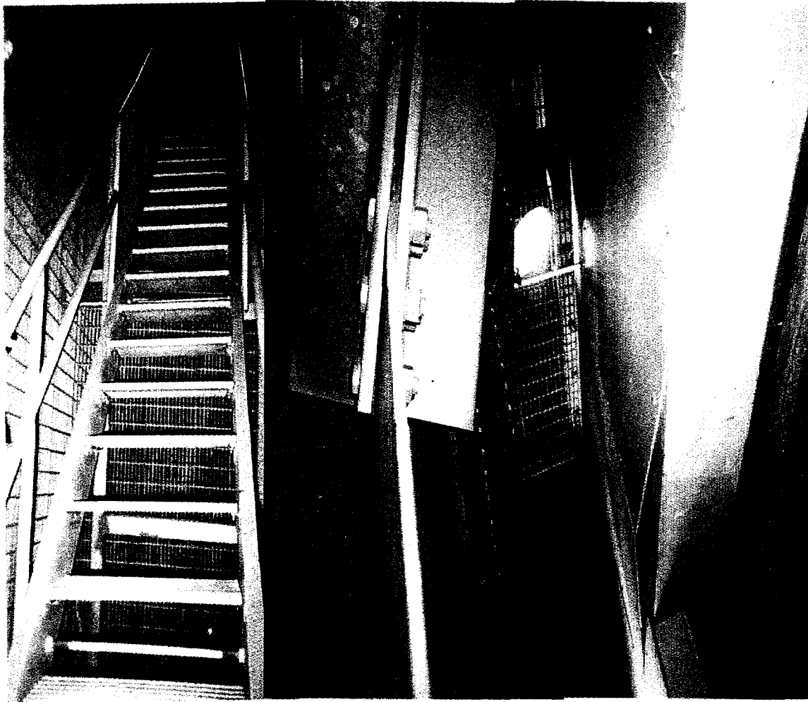
Figure 5. Bent stair rail, bent steel member and cracked steel joint, and buckled fiberglass panels inside hoist building.
