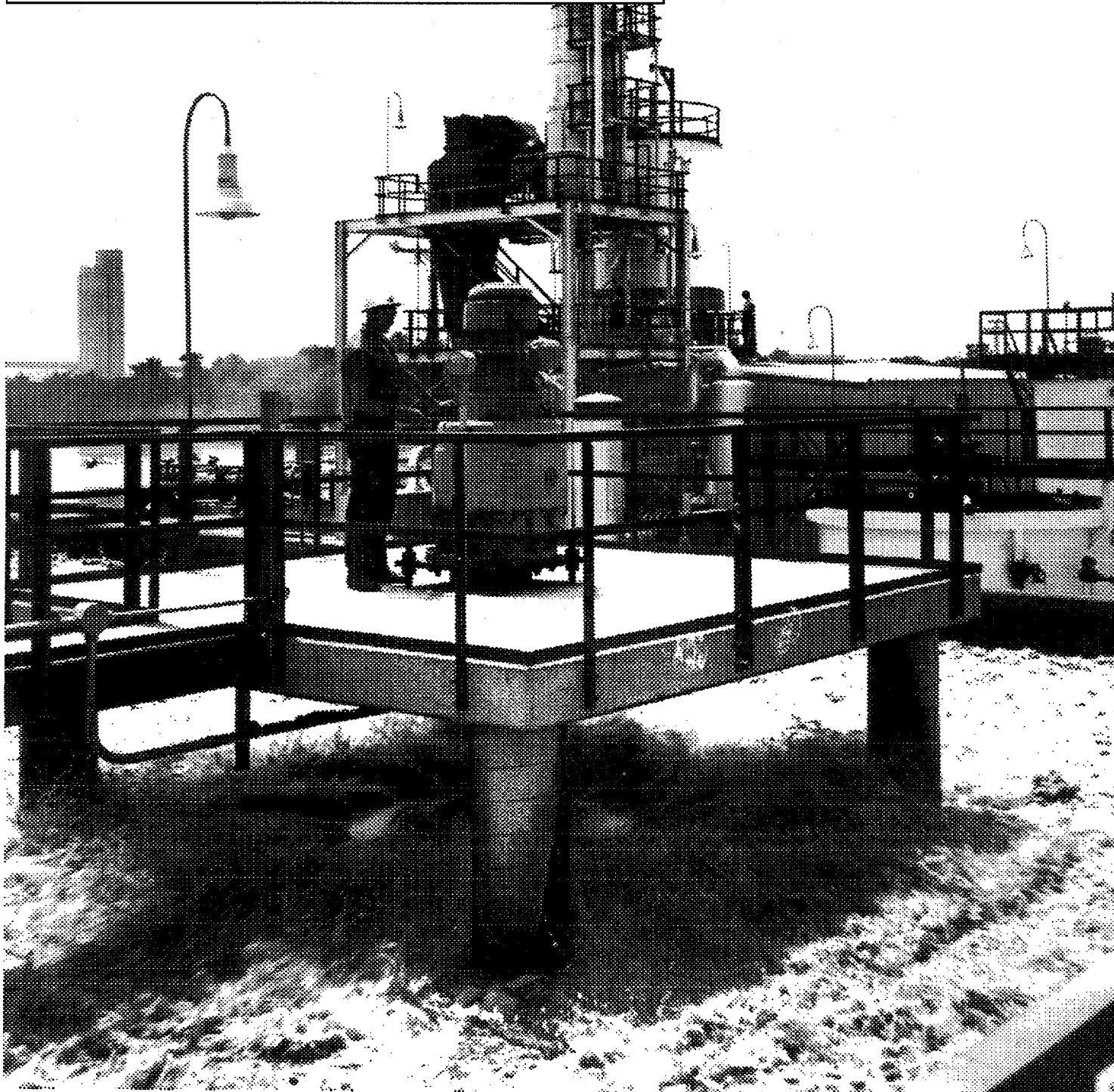
Surface aerators are used at U.S. petroleum refineries to help prevent water pollution. These aerators speed up the oxidation process by beating air into water.
