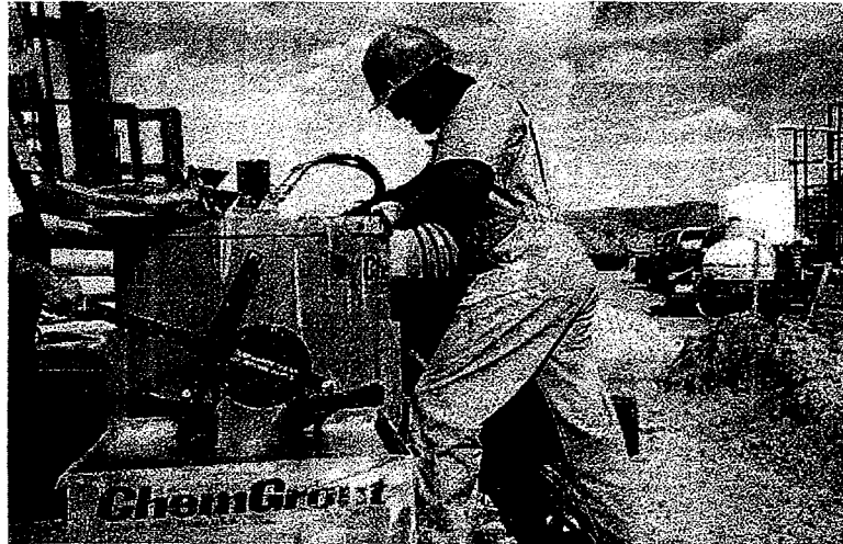
Figure 15. Mixing grout at Sandia. Photo shows grout being transferred from mixing tank to holding hopper.
