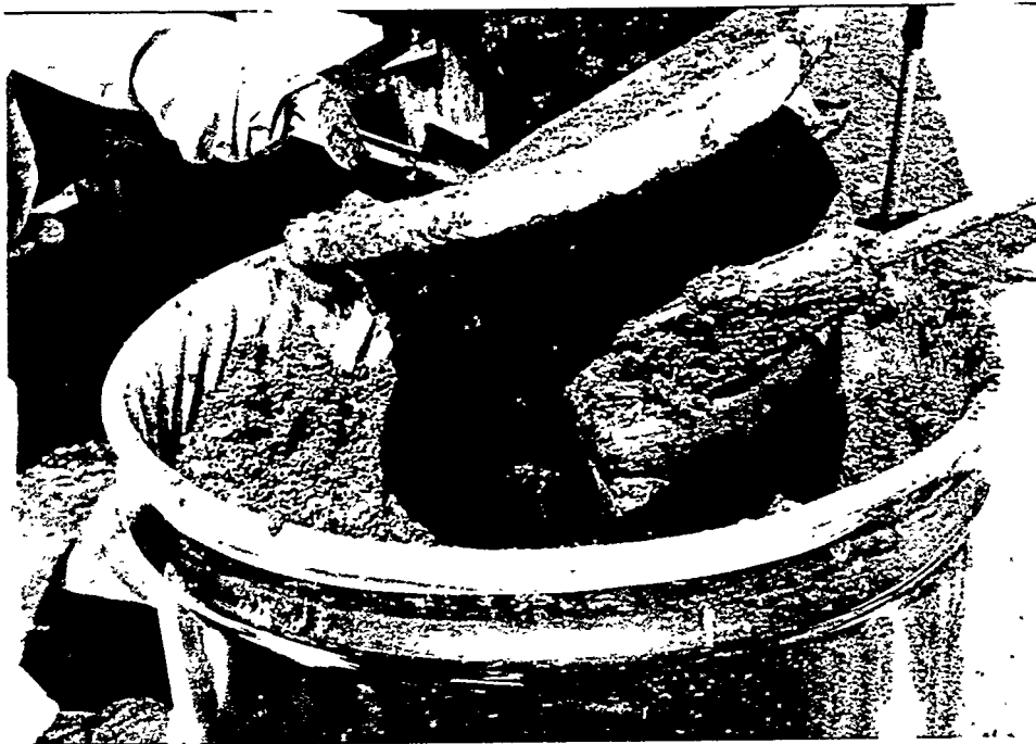
Bitcutter Inside Injection Well source removal August 6, 1996
