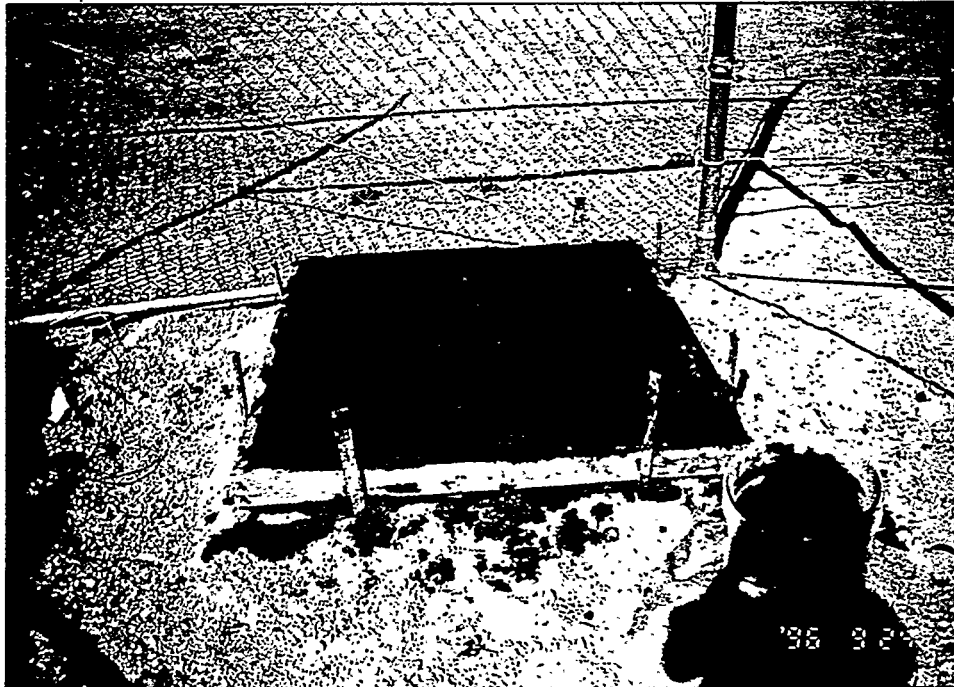
Bitcutter Outside Injection Well concrete cover installation September 24, 1996
