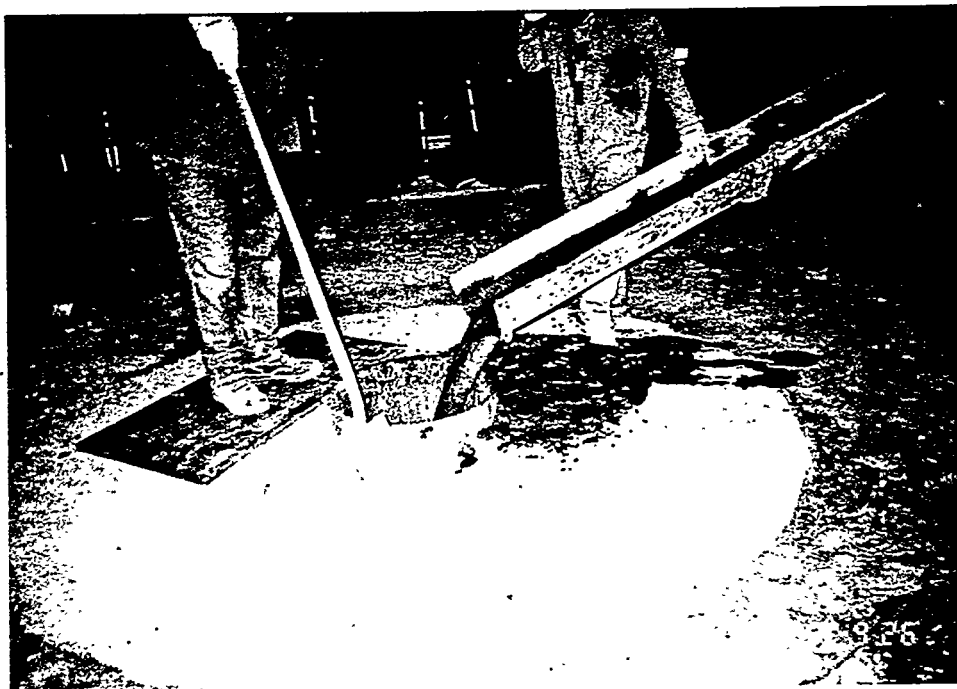
Postshot Containment Shop Injection Well placement of grout plug September 26, 1996
