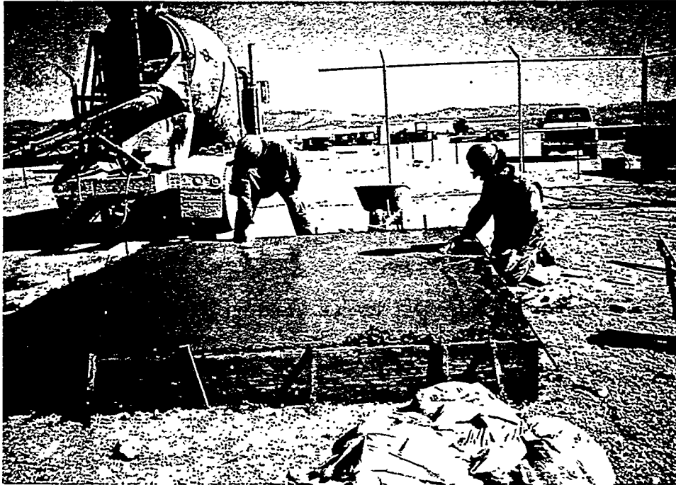
Bitcutter Inside Injection Well concrete cover installation September 24, 1996
