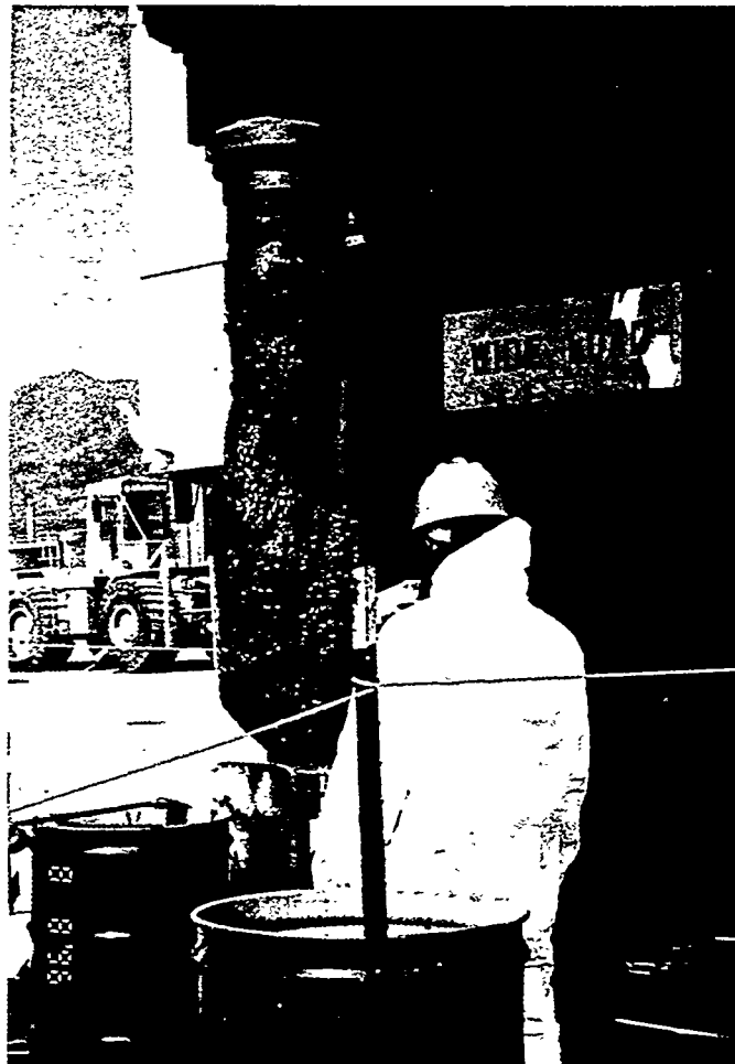
Postshot Containment Shop Injection Well source material removal August 8, 1996
