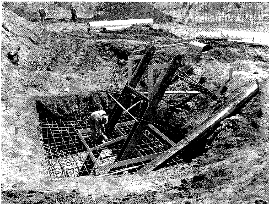
Fig. 3.5 Typical Guy Anchor under Construction.
