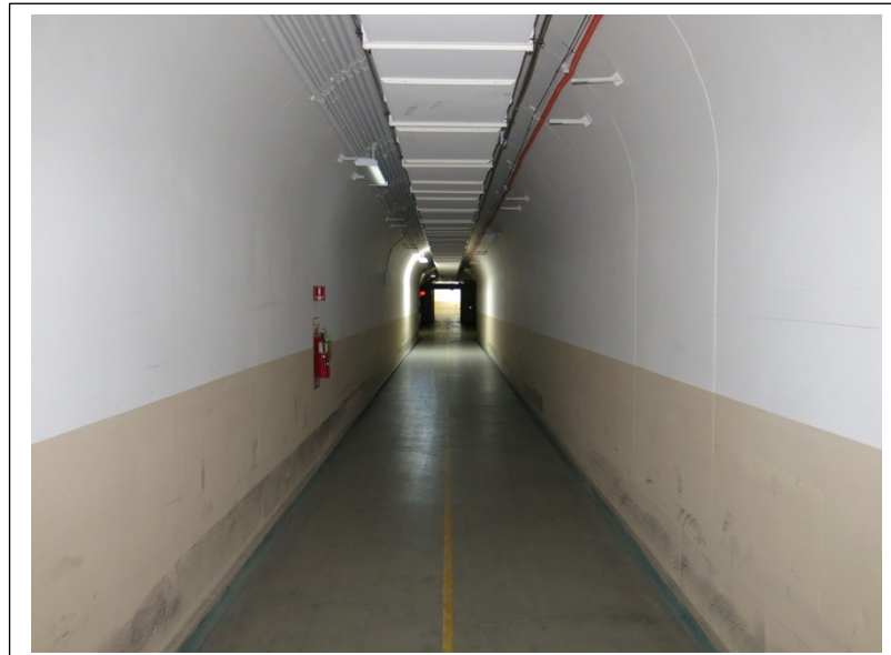
Figure 4. A hallway in the Manzano Mesa MP-1 underground complex.
