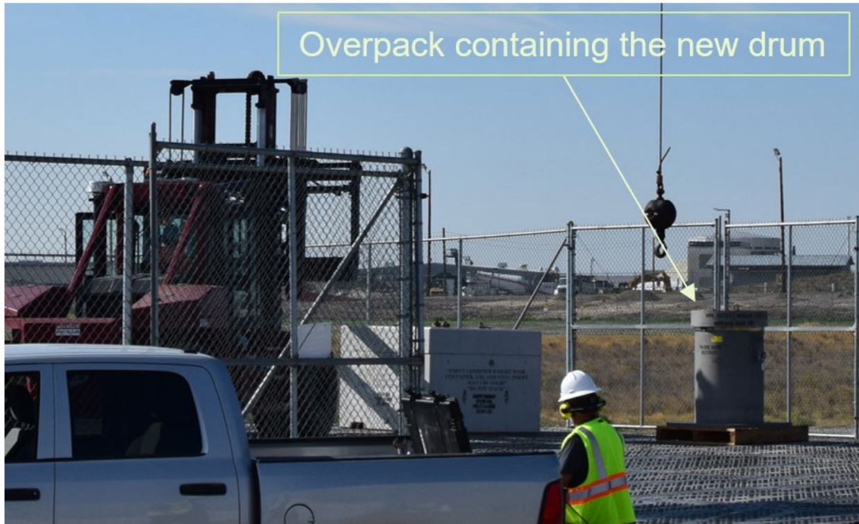
Figure 14. Positioning of the ISC at the staging area next to the overpack containing the new drum.
