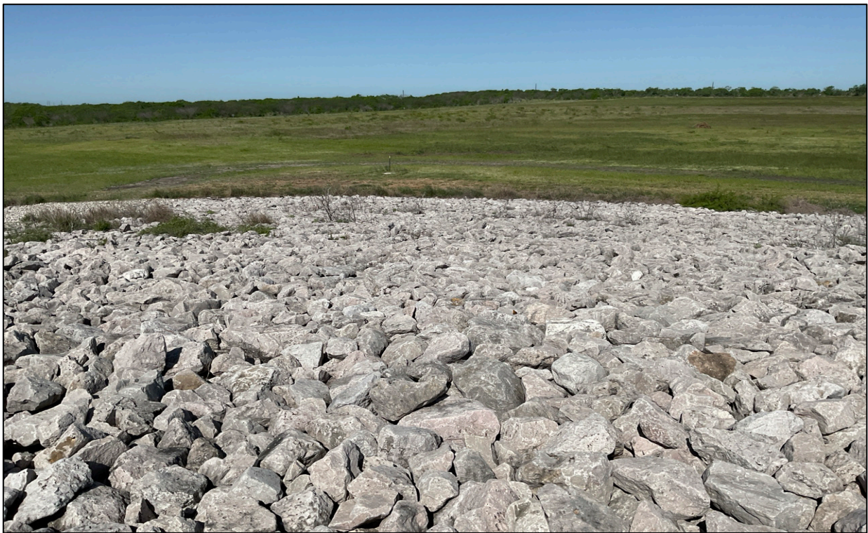
PL-6. Vehicle Tracks on West Slope of Disposal Cell
