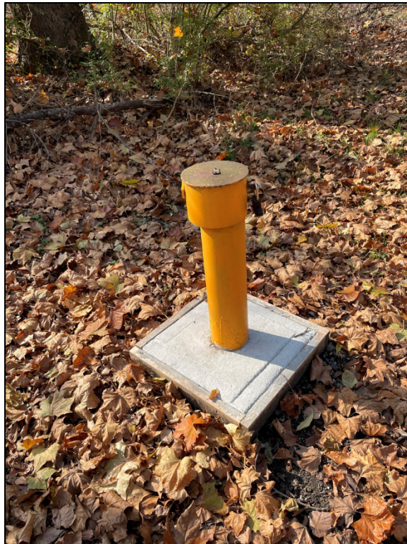
PL-4. New Well Pad at Well 0424
