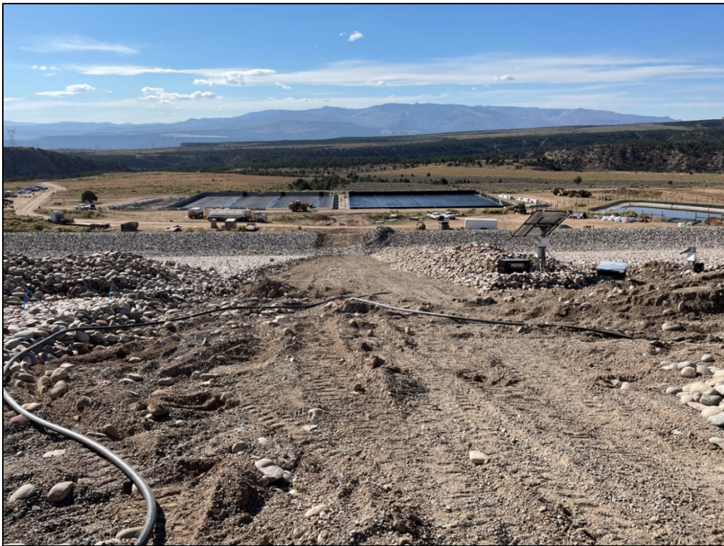
PL-6. Newly Installed Modular Tanks and Construction Overview
