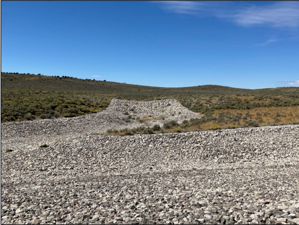
PL-5. Diversion Channel No. 2
