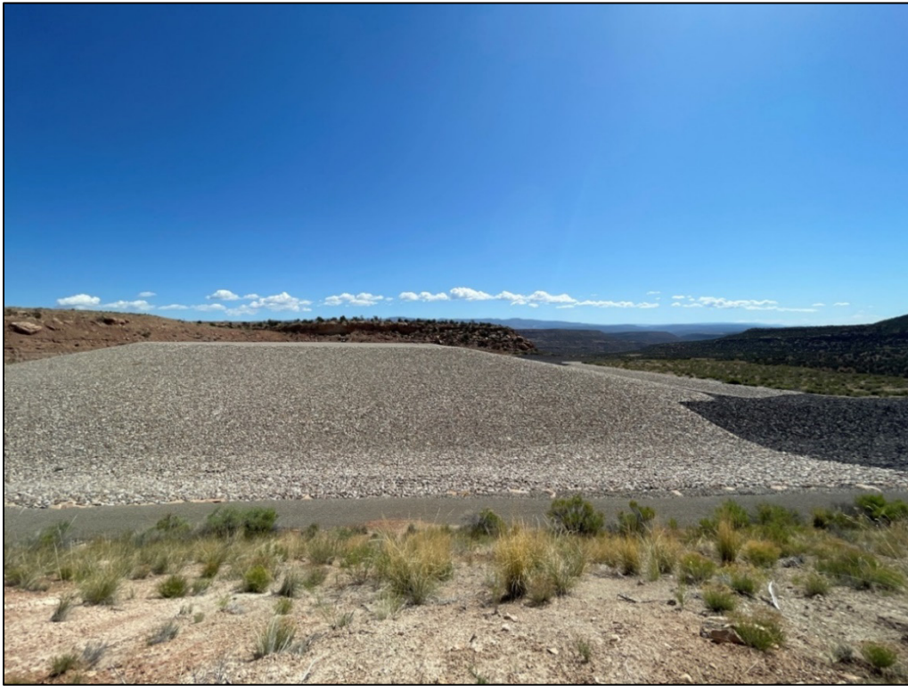
PL-5. Disposal Cell
