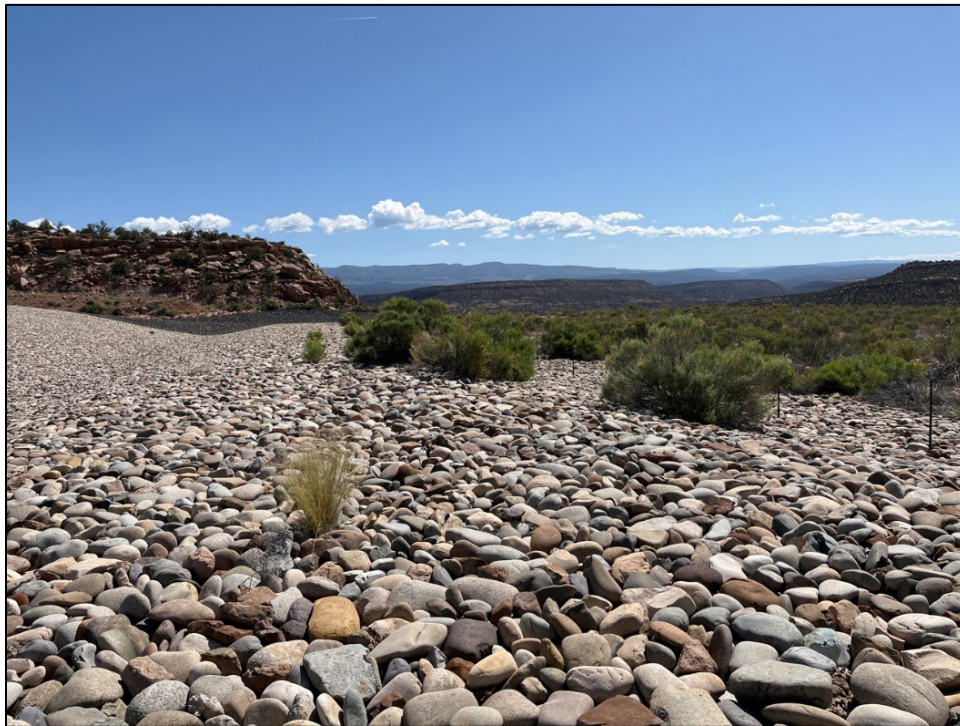
PL-10. Woody Vegetation Growth on Southeast Slopes of Disposal Cell
