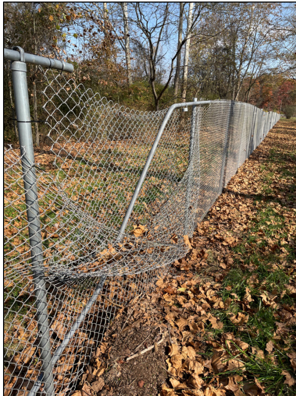
PL-2. Temporary Fence Repair
