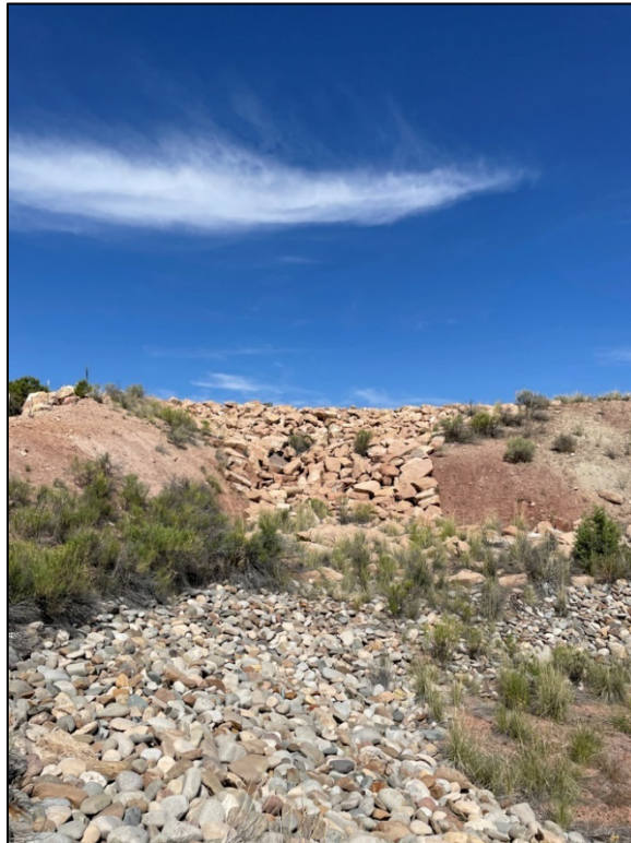
PL-7. Rocks in Spillway
