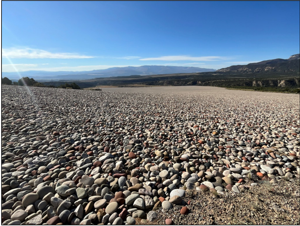
PL-7. Disposal Cell Overview
