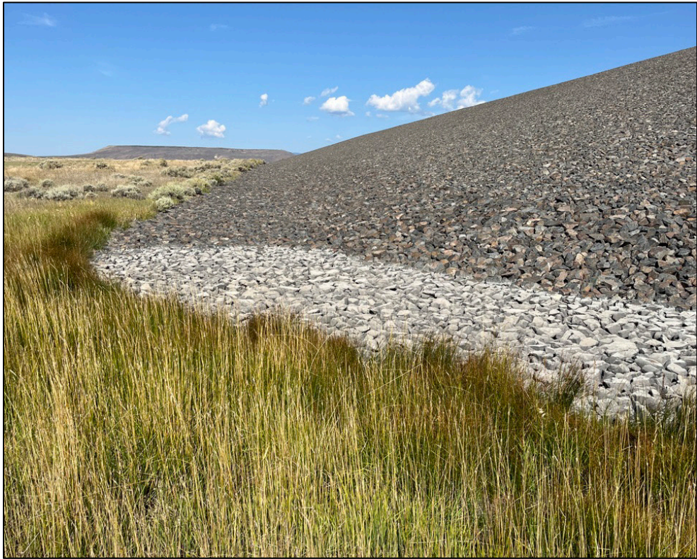
PL-7. Ponding from Stormwater Runoff
