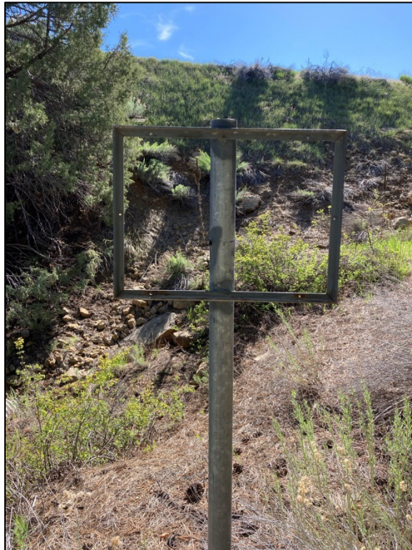
PL-3. Perimeter Sign P82 Missing
