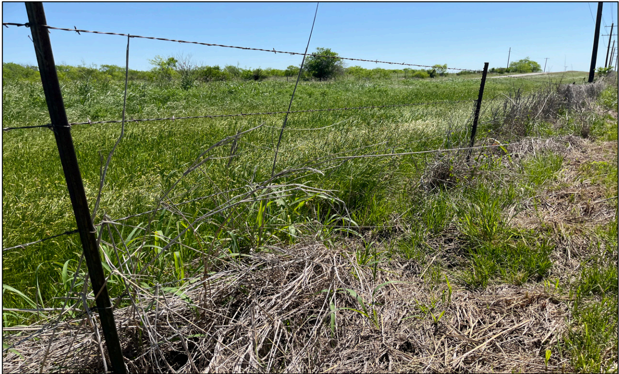
PL-1. Damaged Fence Line
