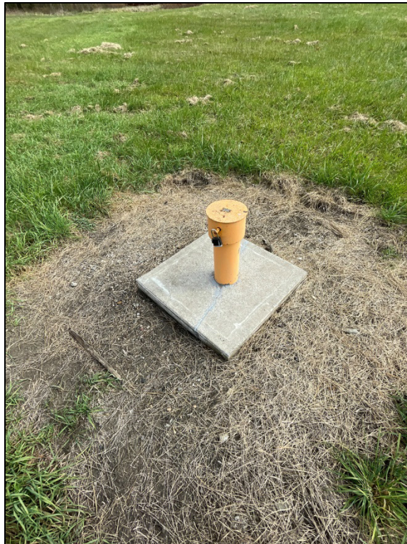
PL-6. Crack Repaired at Well Pad of Monitoring Well 0422
