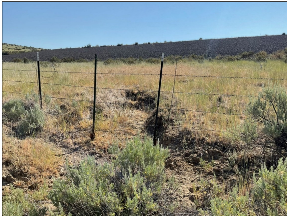
PL-9. Headcutting at Apron Toe Drain 3
