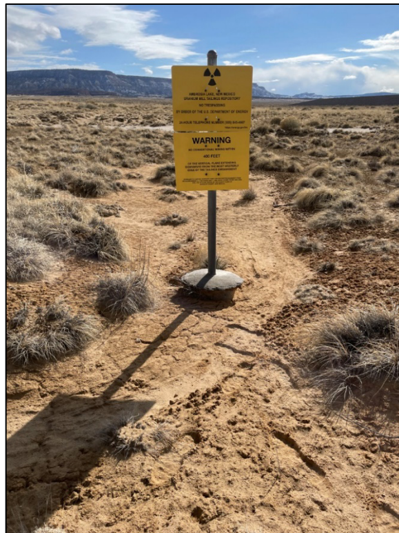
PL-2. Perimeter Sign P12 with Wind Erosion at Base (Stable)
