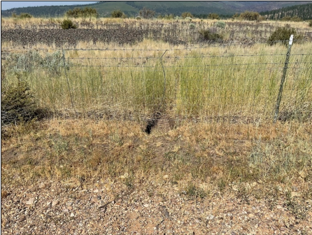
PL-3. Animal Digging Under Eastern Fence Line
