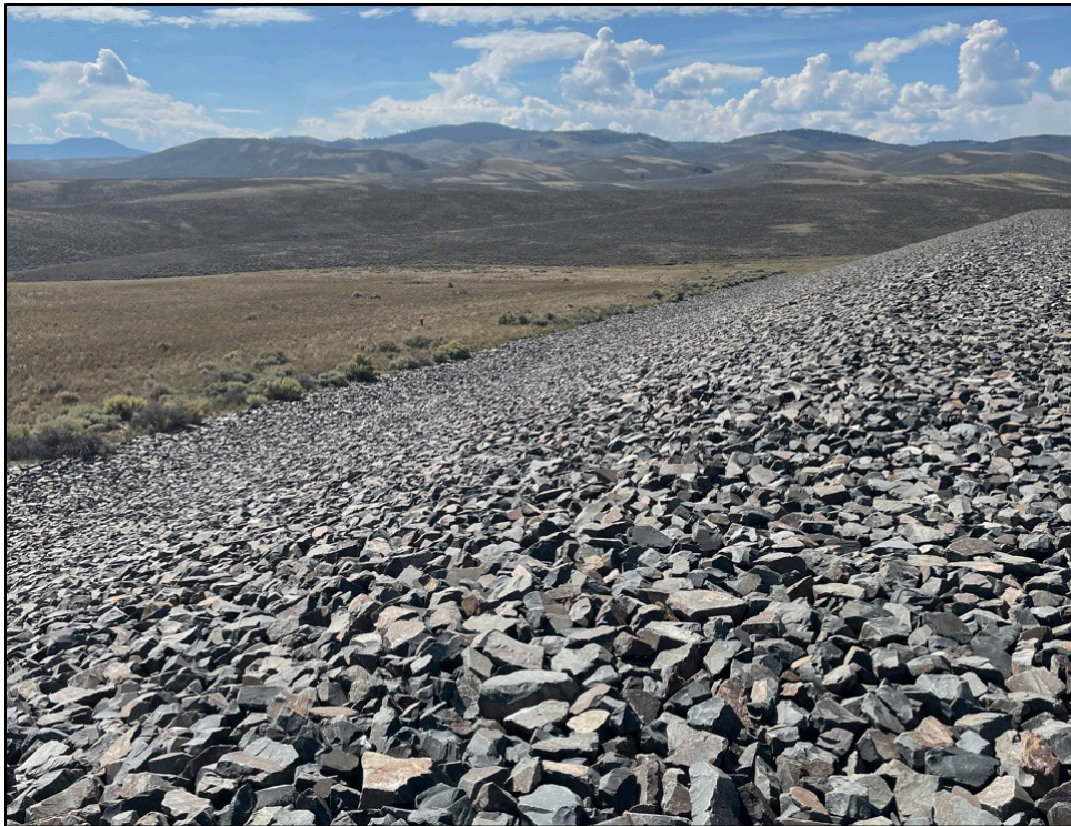
PL-6. East Side Slope
