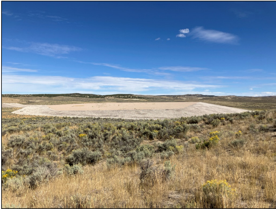
PL-3. Disposal Cell Overview
