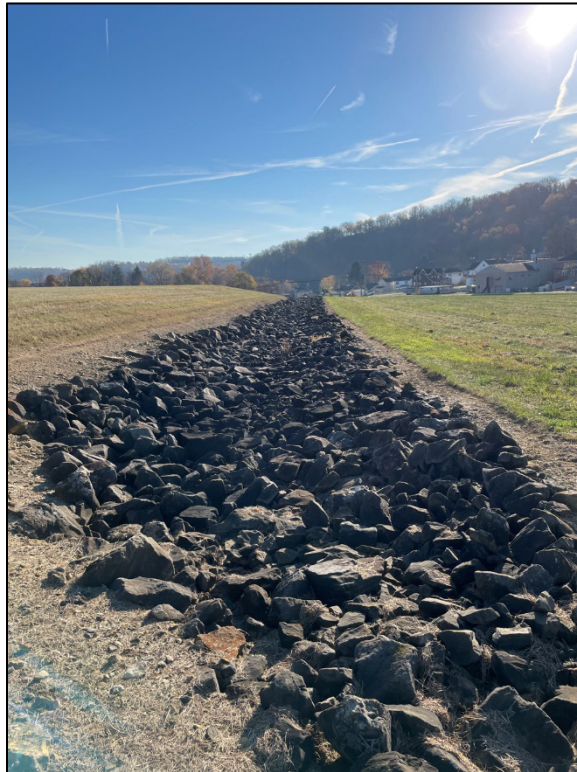
PL-5. Riprap-Armored Diversion Channel
