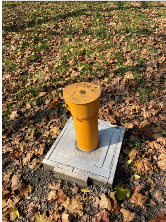
PL-5. New Well Pad at Well 0524
