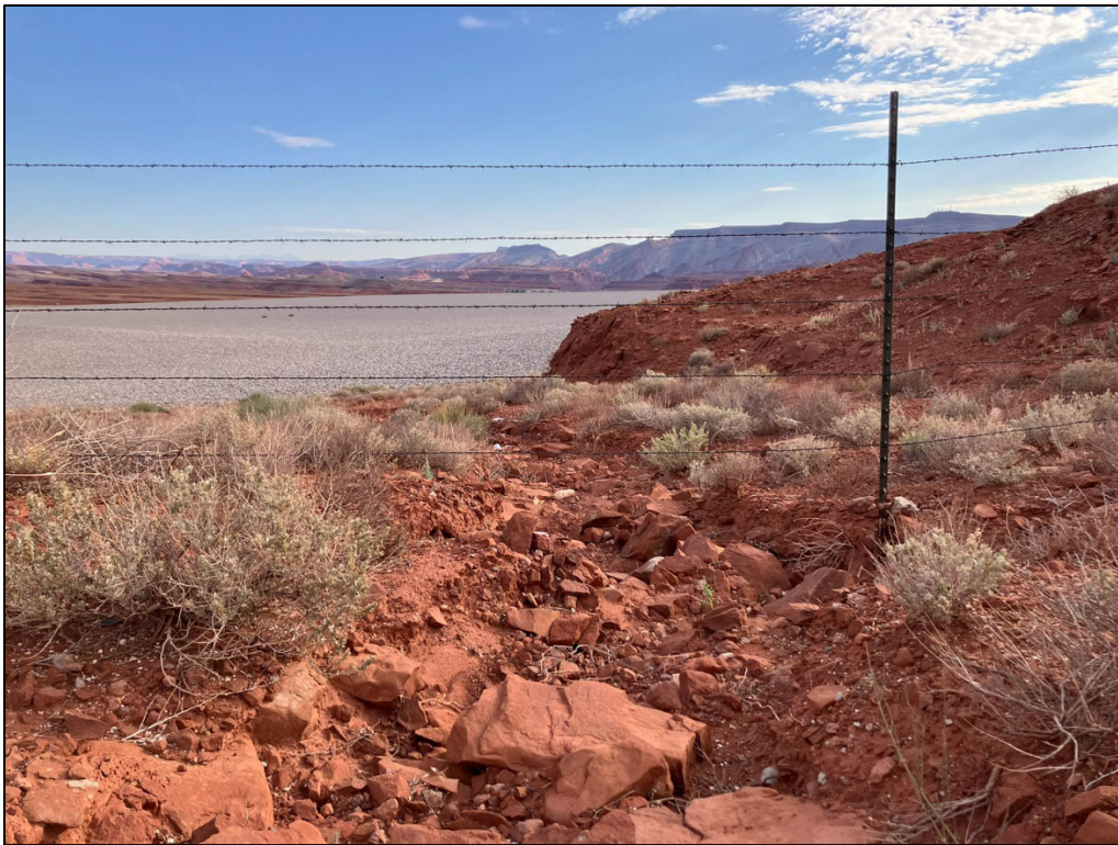
PL-2. Erosion Under Fence
