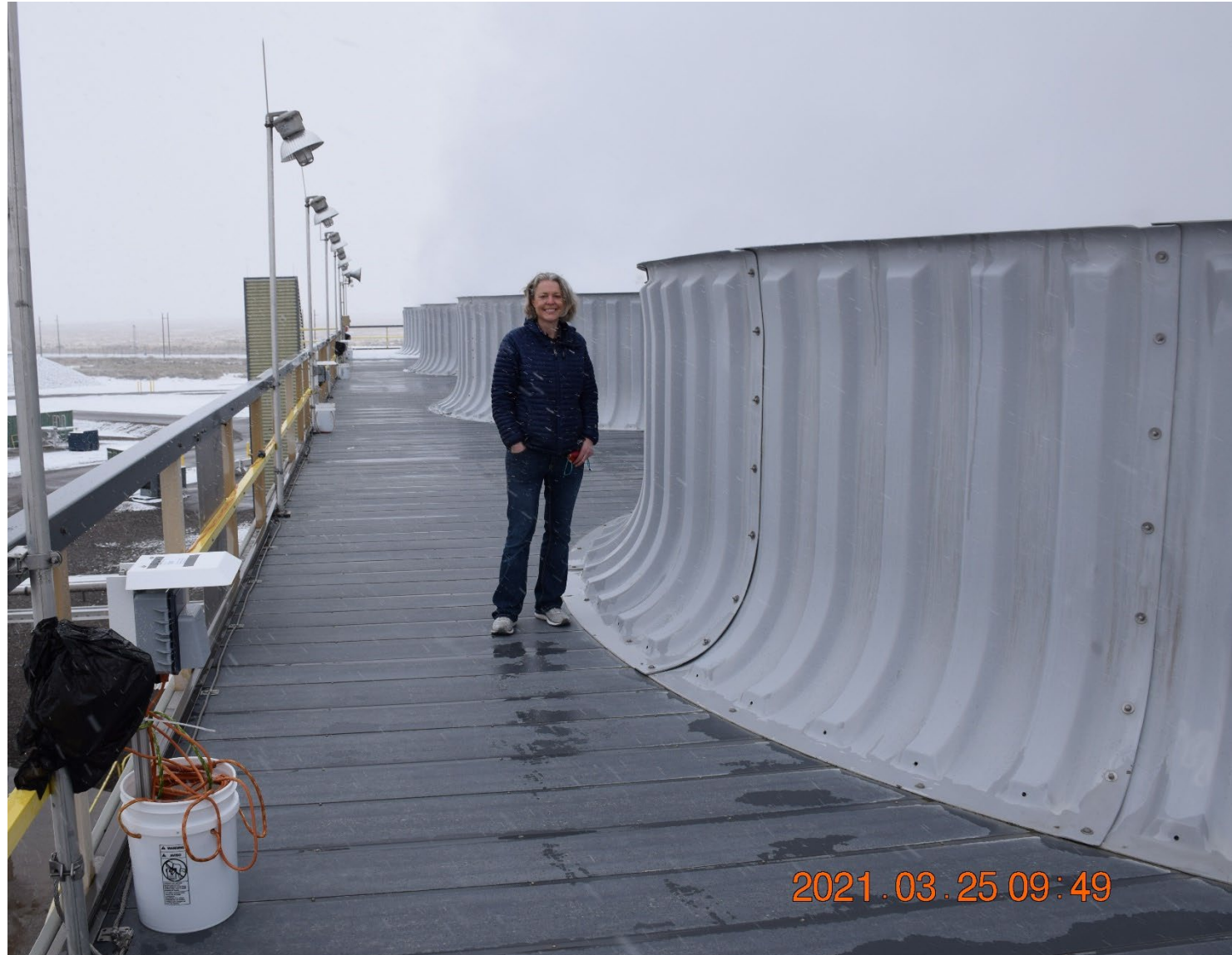
A visit to the deck on the cooling tower
