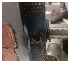
Evidence of high voltage present from high power system test
