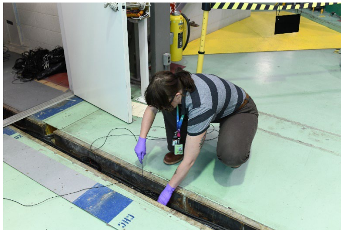
Figure 24. Placement of signal and high voltage cables inside the trench.
