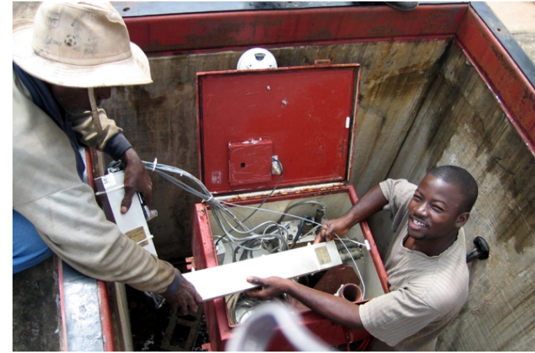
Primary seismic station PS15, Dimbroko, Cote d'Ivoire.
