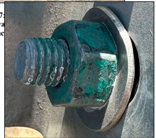
Image 8: Example of bending of washer mounted on an oversized slot.
