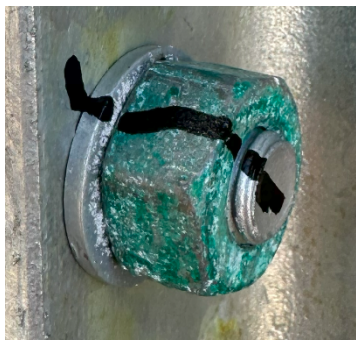
Image 23: Torque stripes detect whether self-loosening has occurred after installation.
