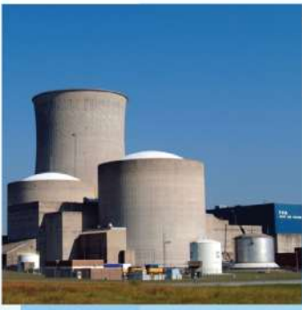
Power uprates and plant life extension
