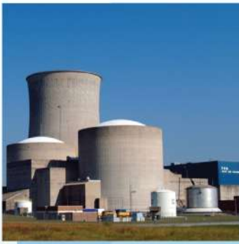
Power uprates and plant life extension
