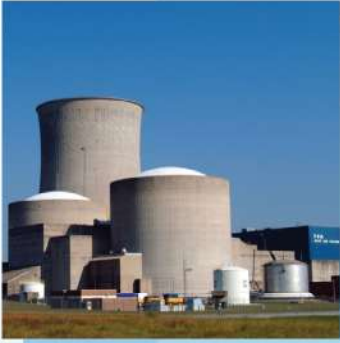
Power uprates and plant life extension
