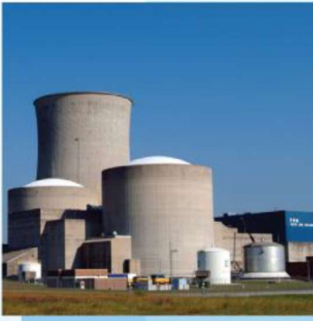
Power uprates and plant life extension
