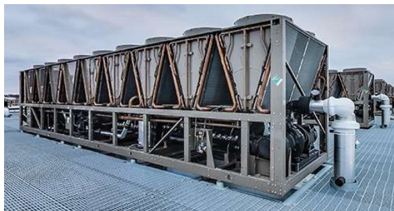
Figure 15: Large Rooftop Chiller Unit for Data Center [20].
