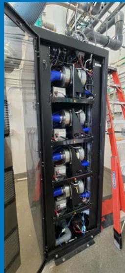
(b) Fuel cell stack setup
