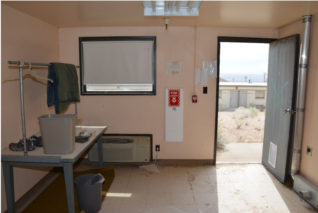
DRI Photo 7: 2531_1582. Room 47, public laundry room interior. Elevation: NA Direction facing: East Photographer: DRI Date: April 17, 2025
