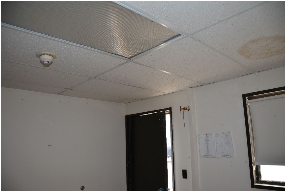
DRI Photo 9: 2531_1545. Room 1, standard bedroom interior, ceiling detail. Elevation: NA Direction facing: Detail Photographer: DRI Date: April 17, 2025
