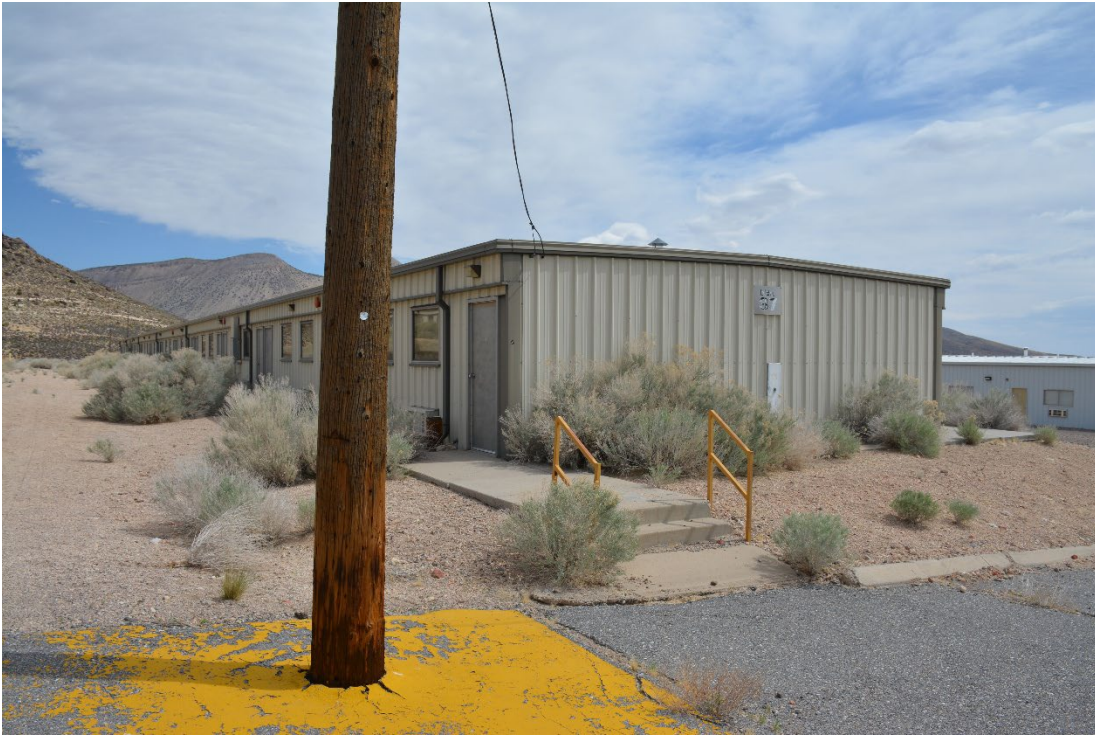
DRI Photo 1: 2531_1598. Overview of the west and south elevations, current condition. Elevation: West/South Direction facing: Northeast Photographer: DRI Date: April 17, 2025
