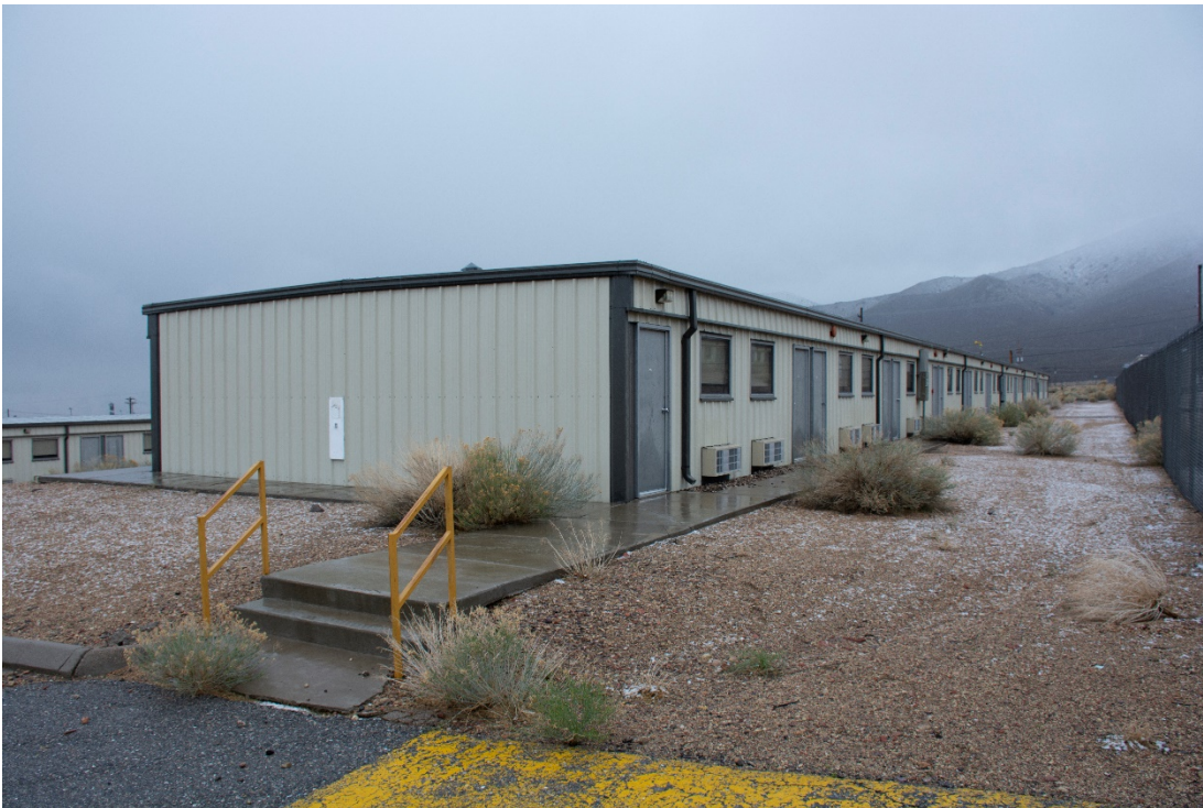
DRI Photo: DSC_4614. Oblique view - north and west elevations. Elevation: North/West Direction facing: Southeast Photographer: DRI Date: March 23, 2020
