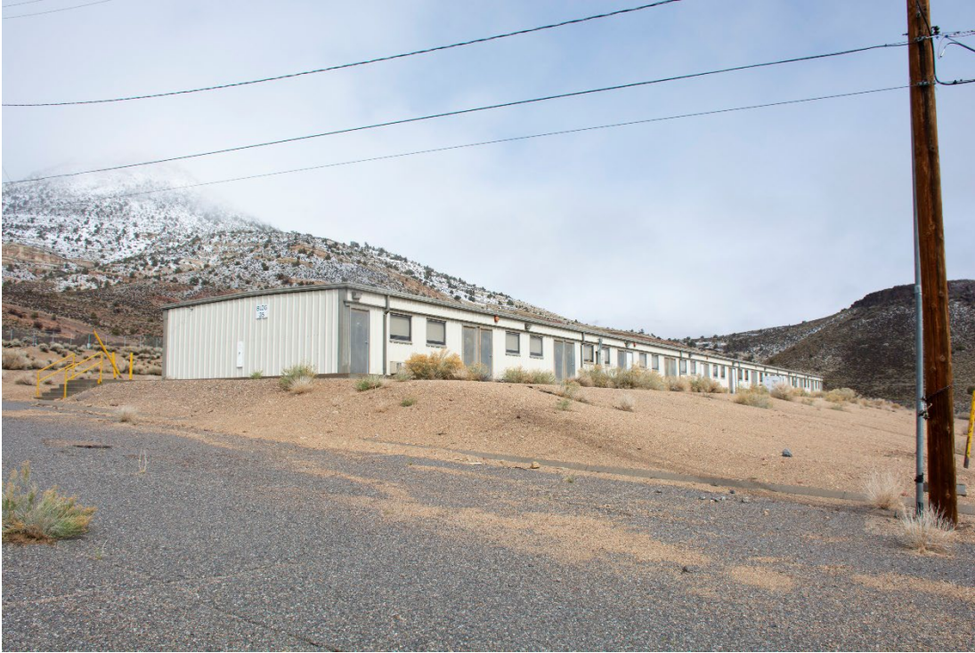
DRI Photo: DSC_4688. Oblique view - south and east elevations. Elevation: South/East
