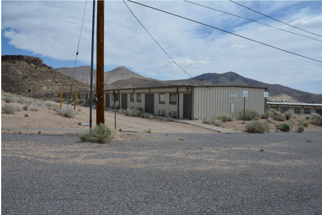
Figure 2: Building 12-34, overview of the west and south elevations (DRI 2531_1595, 2025).
