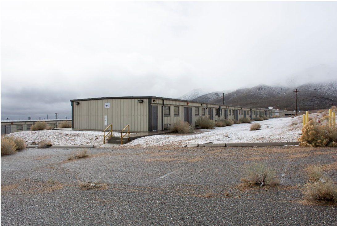
DRI Photo: DSC_4662. Oblique view - north and west elevations. Elevation: North/West Direction facing: Southeast Photographer: DRI Date: March 23, 2020
