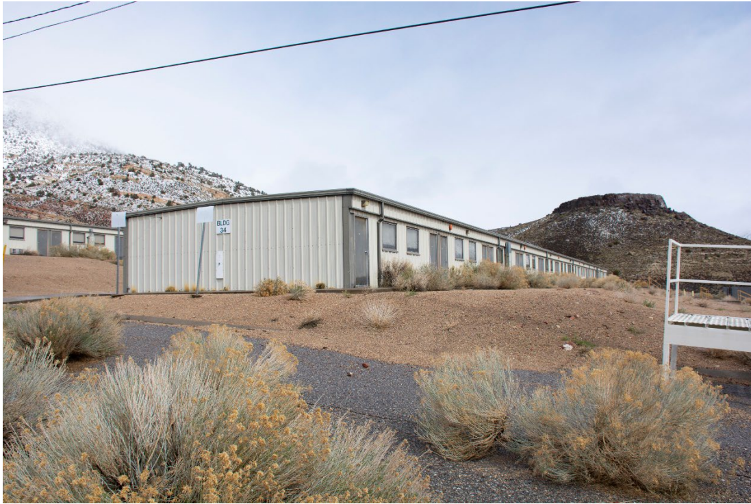
DRI Photo: DSC_4682. Oblique view - south and east elevations. Elevation: South/East Direction facing: Northwest
