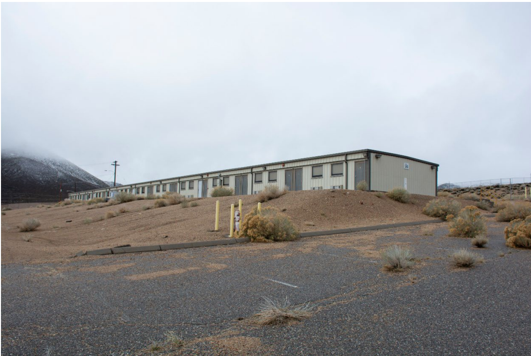
DRI Photo: DSC_4708. Oblique view - east and north elevations. Elevation: East/North Direction facing: Southwest Photographer: DRI Date: March 23, 2020
