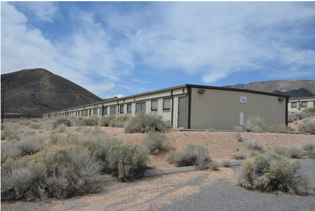
DRI Photo 2: 2531_1605. Overview of the east and north elevations, current condition. Elevation: East/North Direction facing: Southwest Photographer: DRI Date: April 17, 2025
