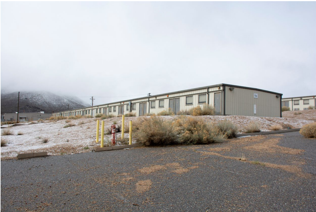
DRI Photo: DSC_4666. Oblique view - east and north elevations. Elevation: East/North Direction facing: Southwest Photographer: DRI Date: March 23, 2020
