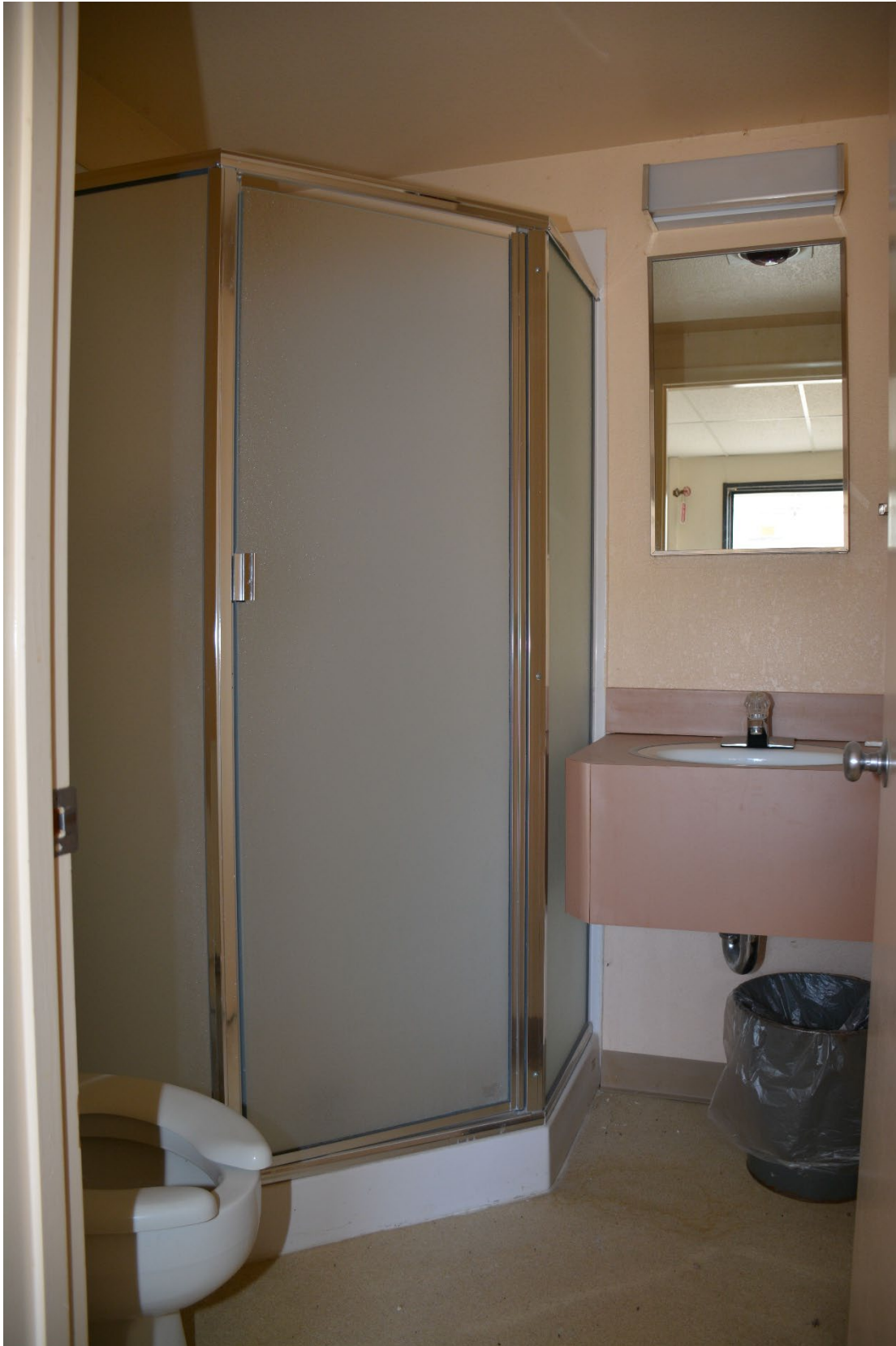
DRI Photo 5: 2531_1540. Room 1, standard bathroom interior. Elevation: NA Direction facing: East-Northeast Photographer: DRI Date: April 17, 2025
