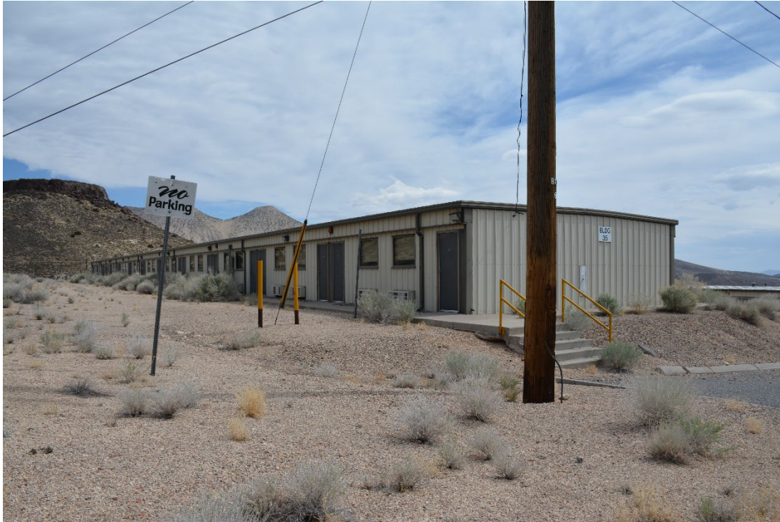
Figure 3: Building 12-35, overview of the west and south elevations (DRI 2531_1592, 2025).
