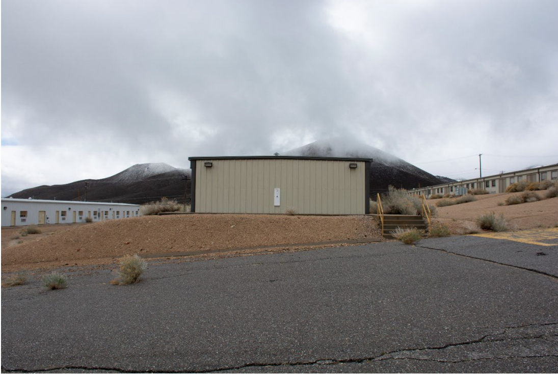
DRI Photo: DSC_4762. North elevation. Elevation: North Direction facing: South Photographer: DRI Date: March 23, 2020
