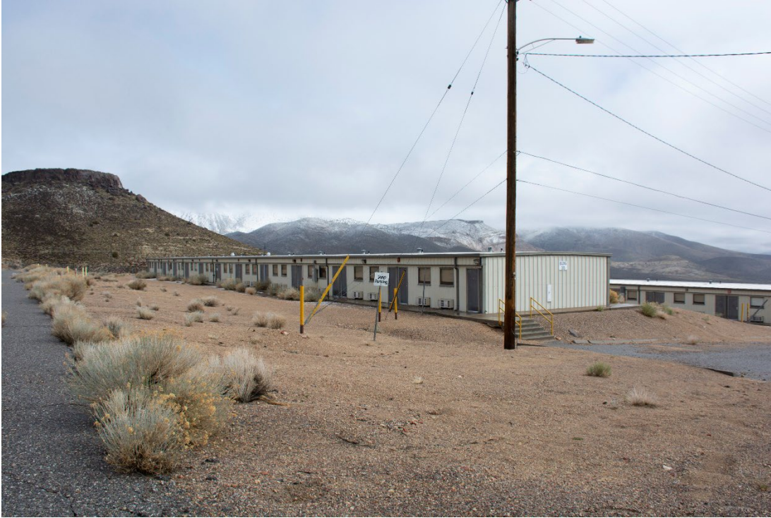
DRI Photo: DSC_4694. Oblique view - west and south elevations. Elevation: West/South Direction facing: Northeast Photographer: DRI Date: March 23, 2020
