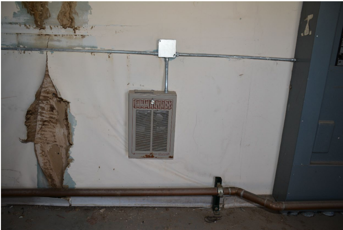
DRI Photo 12: 2531_1619. Room 48, mechanical/equipment room interior, wall heater detail. Elevation: NA Direction facing: East Photographer: DRI Date: April 17, 2025
