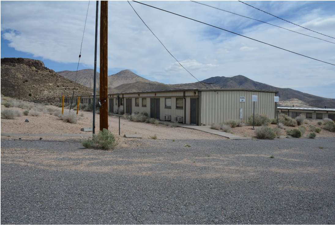
DRI Photo 1: 2531_1595. Overview of the west and south elevations, current condition. Elevation: West/South Direction facing: Northeast Photographer: DRI Date: April 17, 2025
