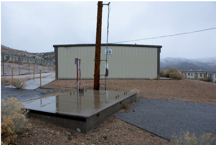
DRI Photo: DSC_4608. AR1 Waste Compactor Foundations.
