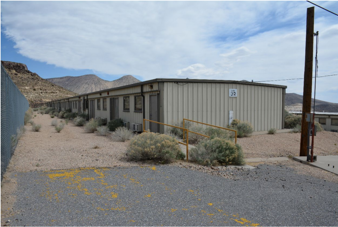
DRI Photo 1: 2531_1596. Overview of the west and south elevations. Elevation: West/South Direction facing: Northeast Photographer: DRI Date: April 17, 2025
