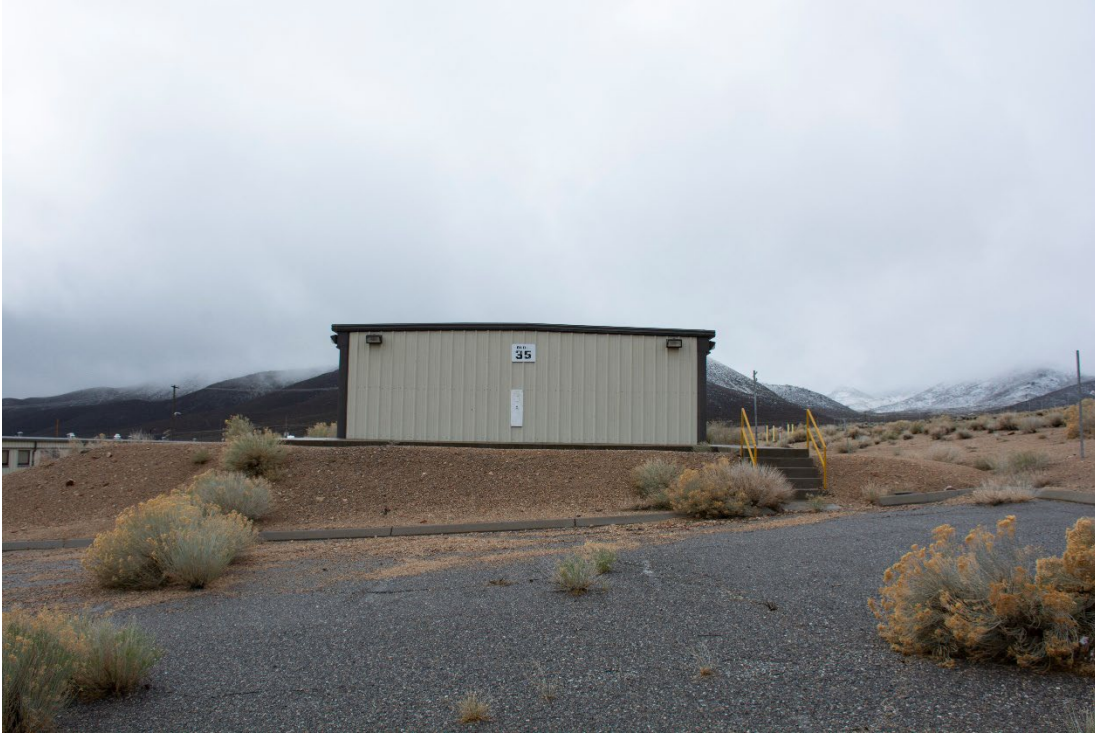
DRI Photo: DSC_4706. North elevation. Elevation: North Direction facing: South Photographer: DRI Date: March 23, 2020
