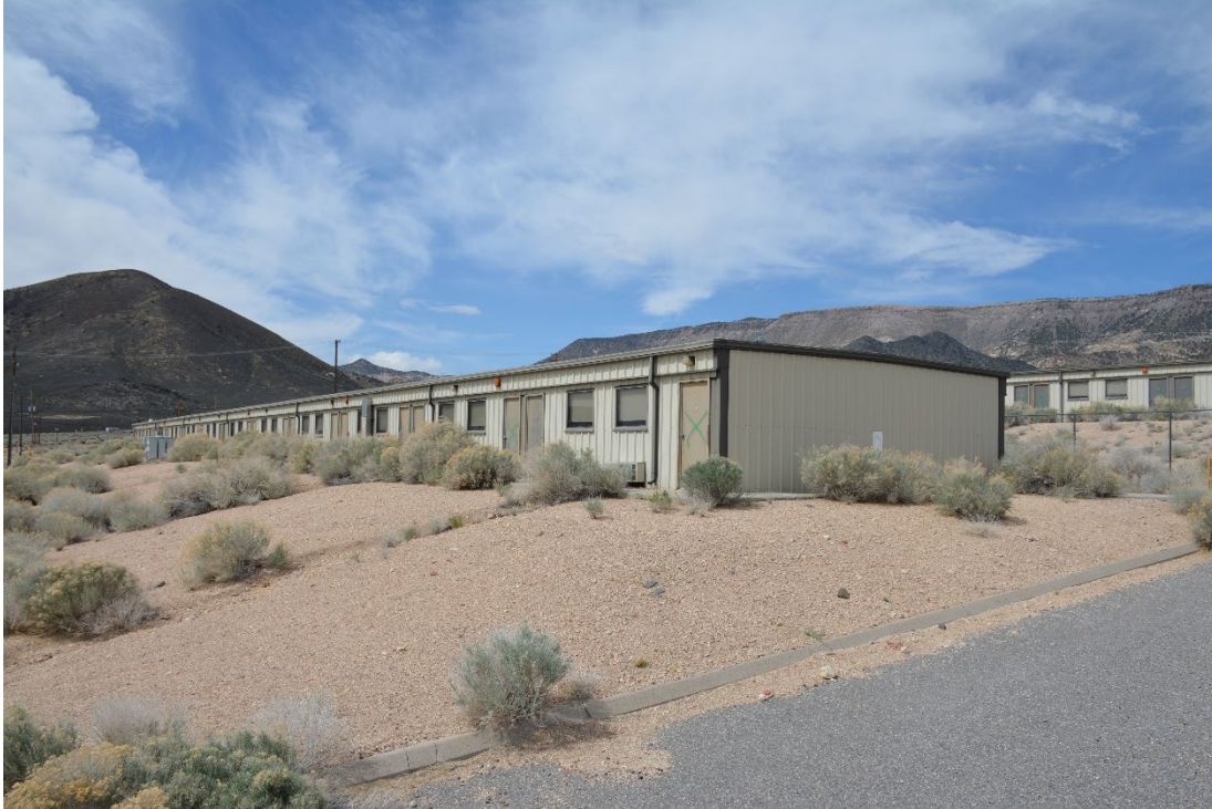
Figure 1: Building 12-32, overview of the east and north elevations (DRI 2531_1602, 2025).
