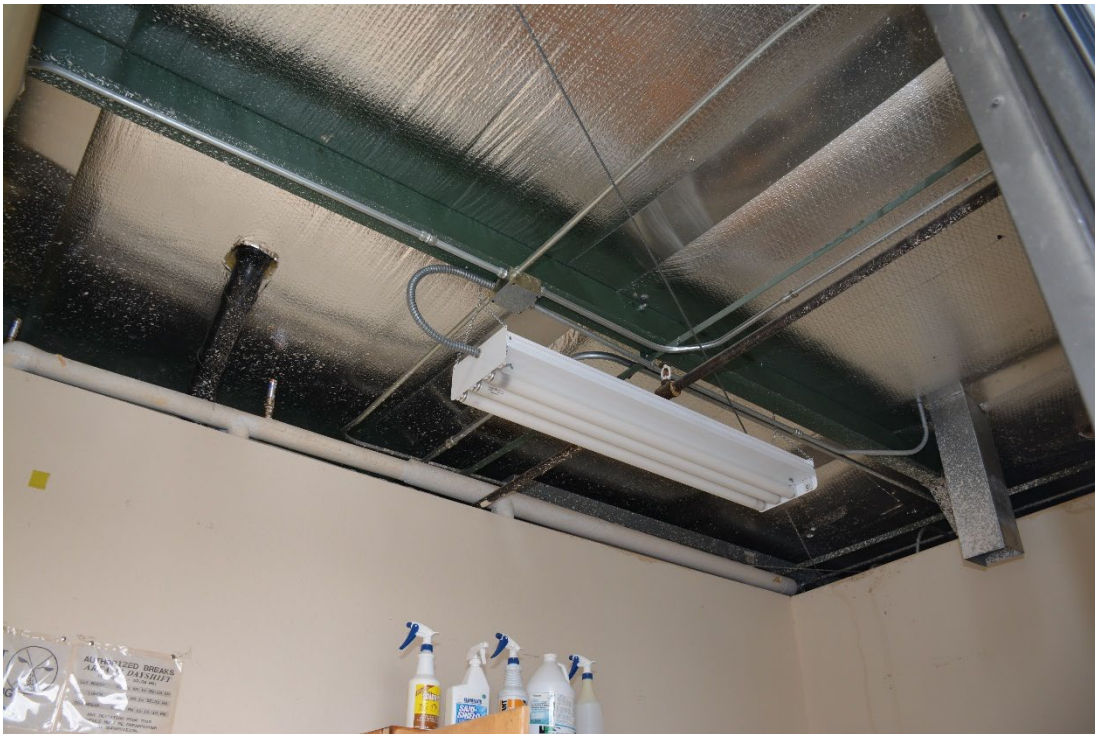
DRI Photo 12: 2531_1565. Room 48, Janitor storage room interior, unfinished ceiling with light fixture, joists, and insulation. Elevation: NA Direction facing: Detail Photographer: DRI Date: April 17, 2025
