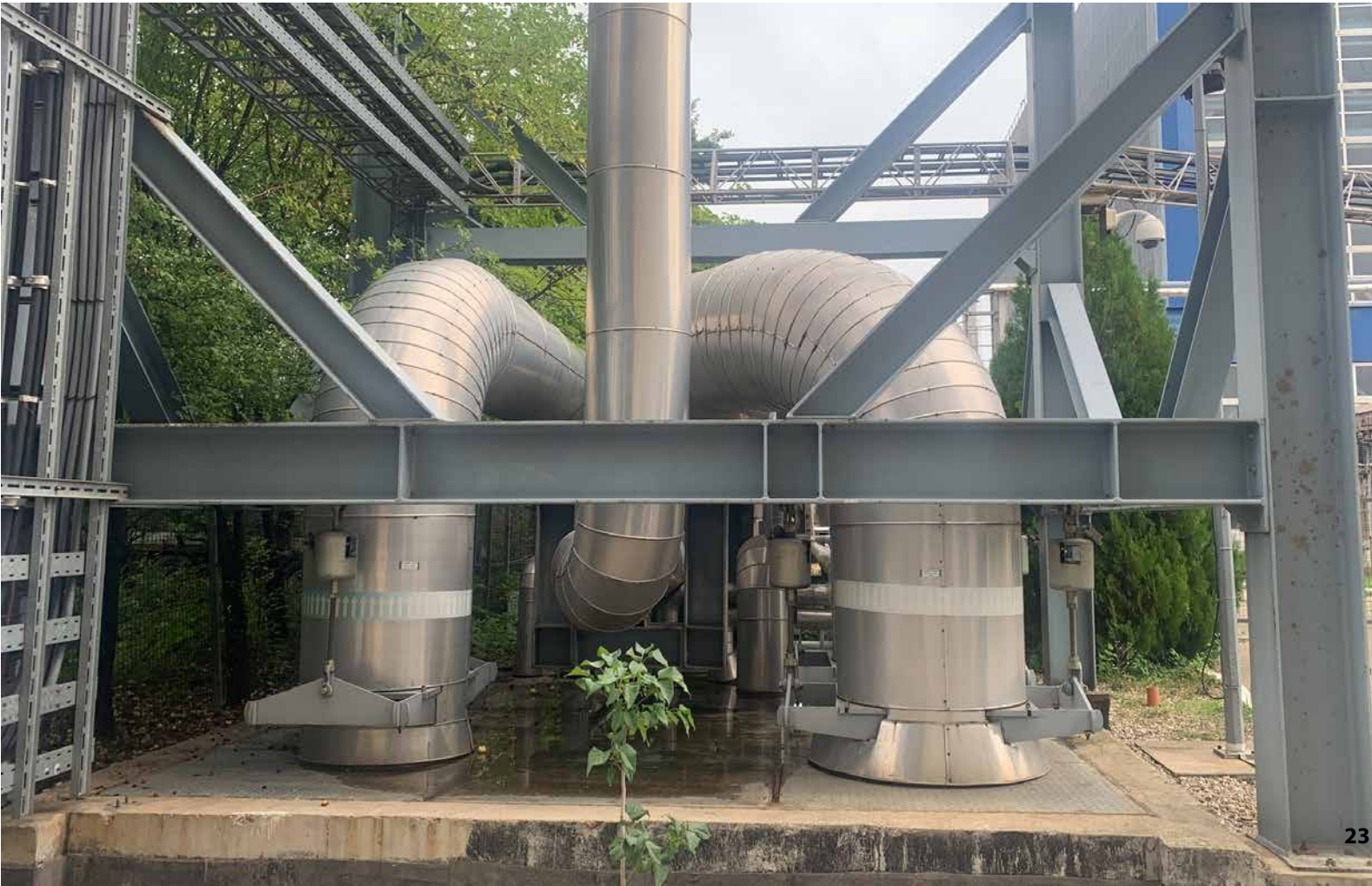
Thermal substation with heat exchangers to buildings. Photo by Shanti Pless, NREL
