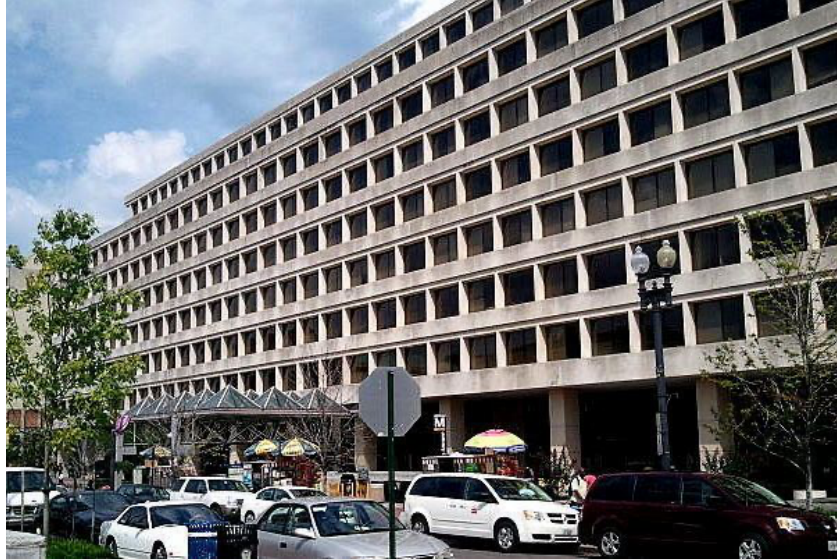
Figure 3-2. One Judiciary Square Building
