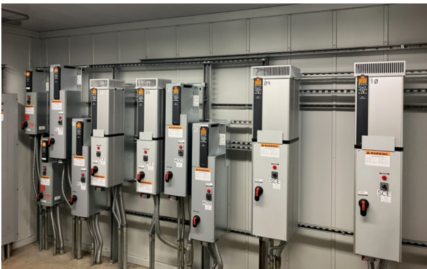
Figure 5: New CEF VFD configuration.
