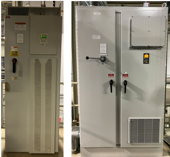
Figure 2: Old VFD (left) and new VFD (right).
